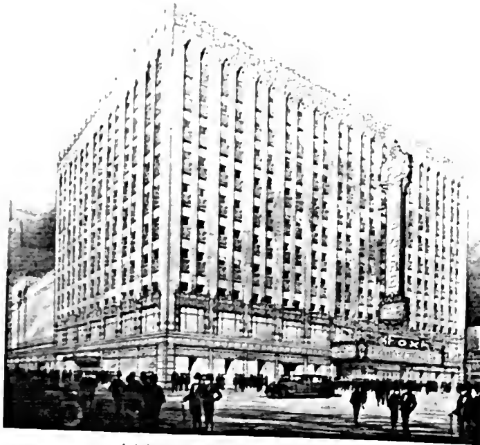
FOX THEATRE AND OFFICE BUILDING, DETROIT
