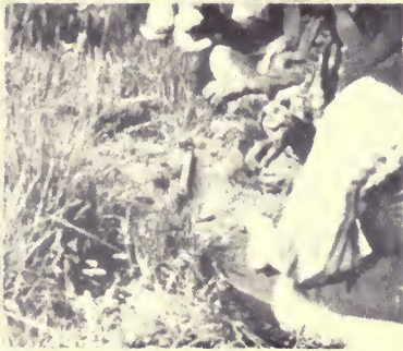
FIG. 19. The pipe-tampers and new earth.
