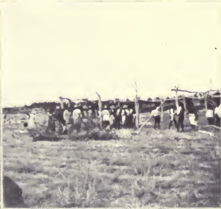
FIG. 44. Erecting the lodge.
