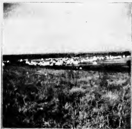
FIG. 2. Section of the camp-circle.
