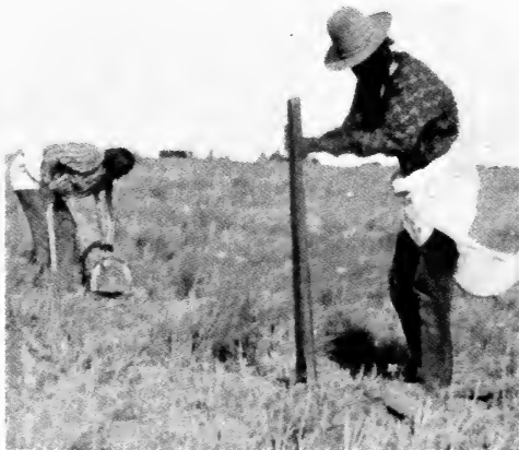
FIG. 46. Digging the hole for the center-pole.
