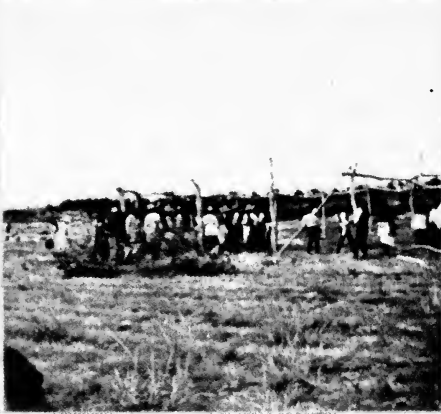
FIG. 44. Erecting the lodge.
