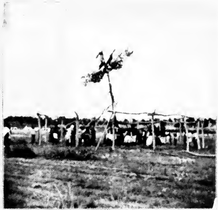
FIG. 54. Raising the center-pole.
