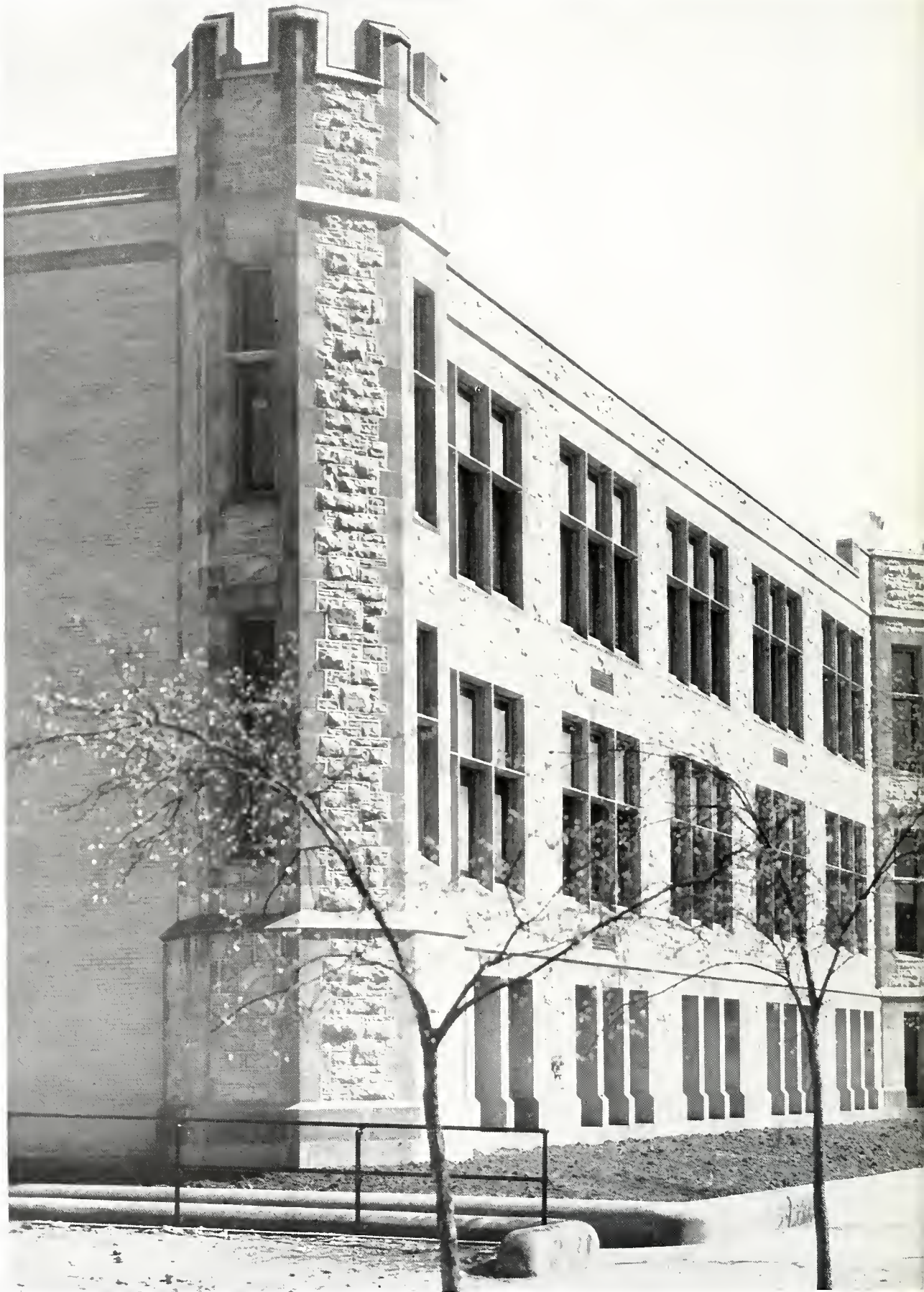
Looking South. Girls' Gymnasium in the Foreground
