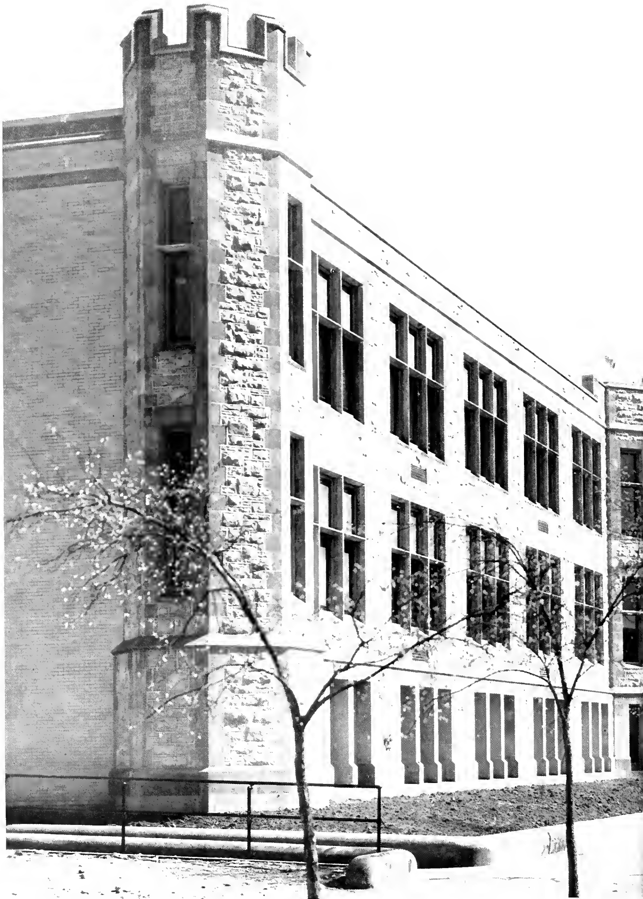
Looking South. Girls' Gymnasium in the Foreground
