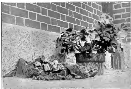
FIG. 26.—An asphalt pavement burst upward by the growth of soft-bodied mushrooms, whose conical heads are visible over the wreckage.
