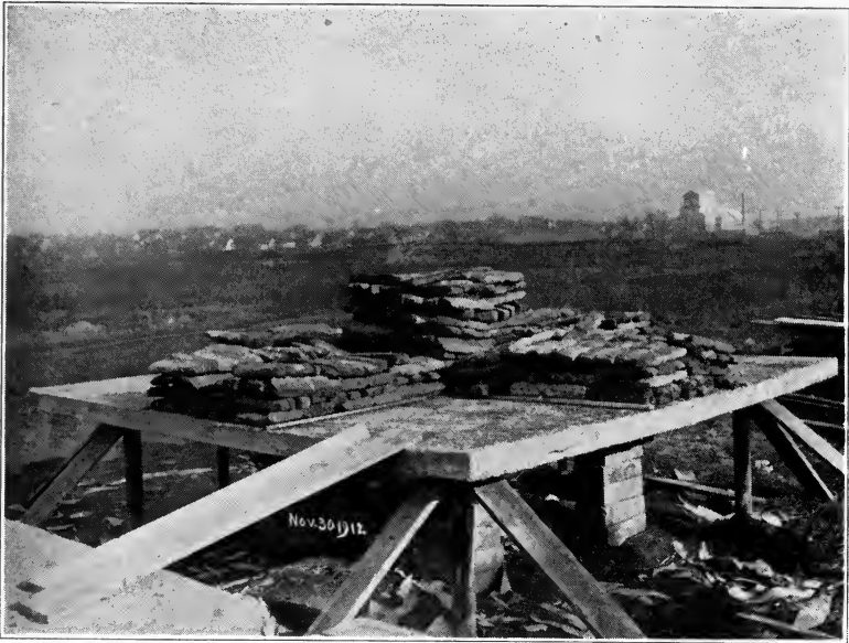
Fig. 8. Norcross Slab Carrying Load 3
