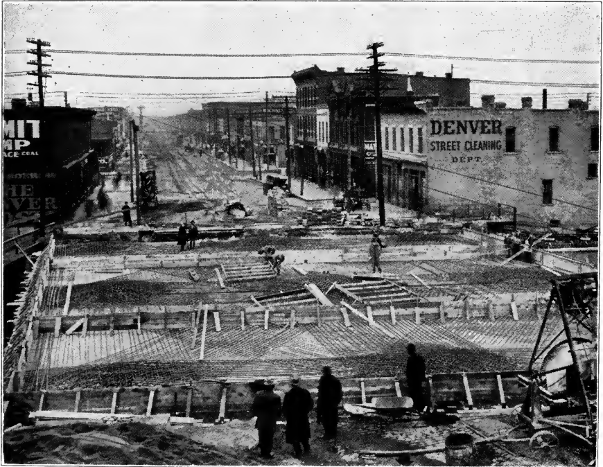
VIEW OF REINFORCING STEEL
