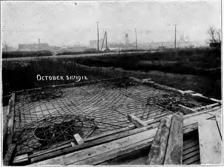
Fig. 12. Reinforcement of Mushroom Slab
