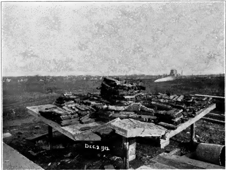
Fig. 10. Collapse of Norcross Slab
