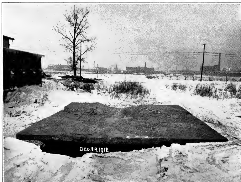
Fig. 19. Failure of Mushroom Slab. Load Removed.
