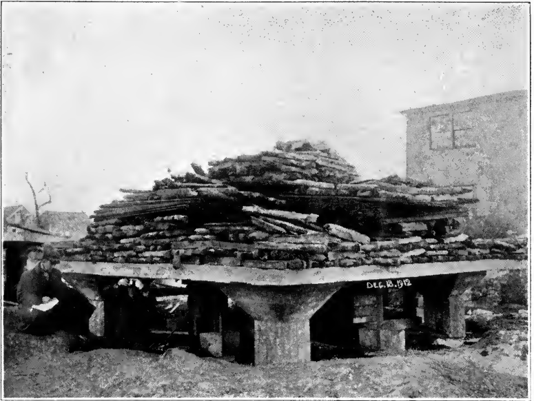
Fig. 15. Mushroom Slab, Load 7.
