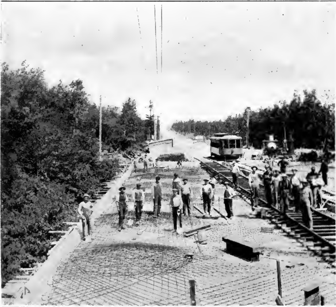
View of Reinforcement in Place TISCHERS CREEK BRIDGE, DULUTH, MINN. Designed by C. A. P. Turner Geo. H. Lounsbury, Contractor
