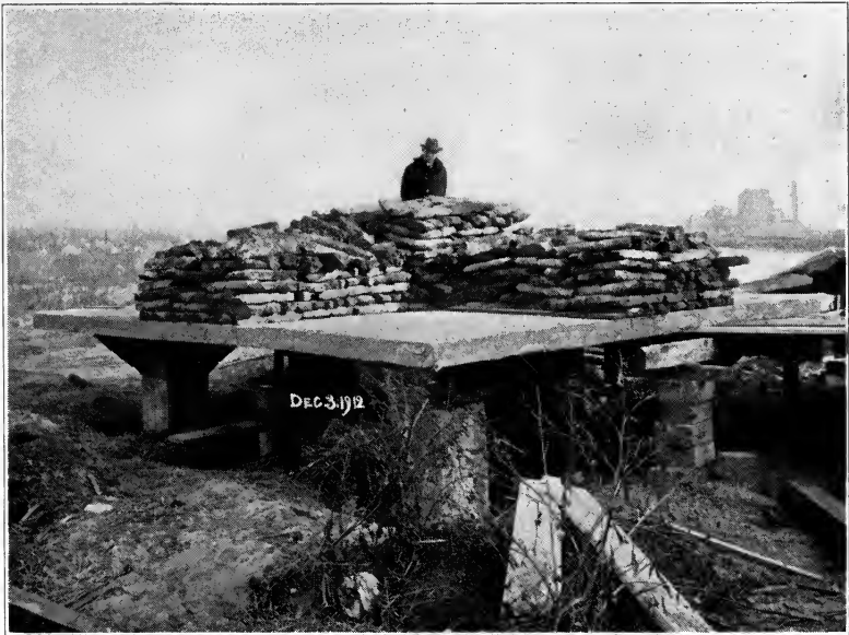
Fig. 14. Mushroom Slab, Load 4.
