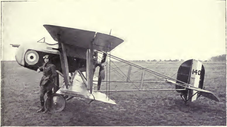
FIG. 116 — 'Vickers Vampire' : Armoured Trench Fighter, fitted with 200 h.p. B.R.2 Engine.
