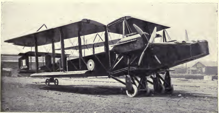
FIG. 3.—Method of folding Back Wings of a large Machine for Storage Purposes.
