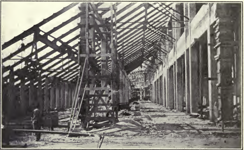
Steel beams (painted with Durable Metal Coating) of the Stadium, Harvard University. Prof. L. J. Johnson, engineer.
