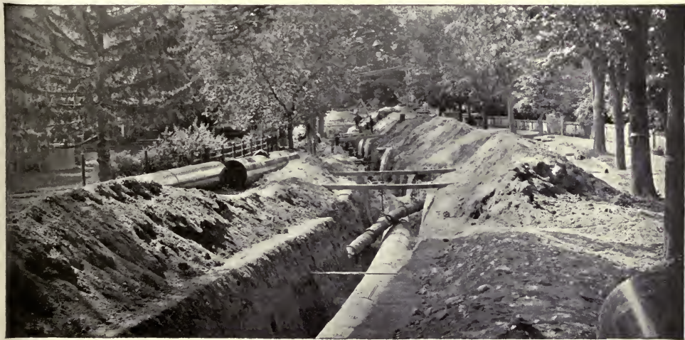
Forty-inch riveted steel pipe, Cambridge, Mass., 1895. Coated with Sabin Pipe Coating.
