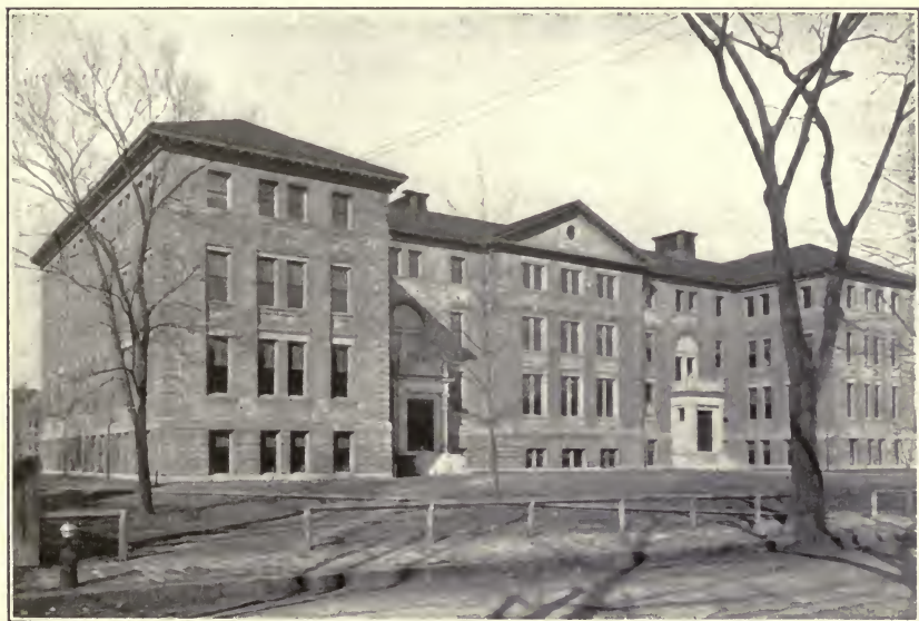
Pierce Hall (Engineering building), Harvard University. Steel framework painted with Durable Metal Coating. Prof. L. J. Johnson, engineer.
