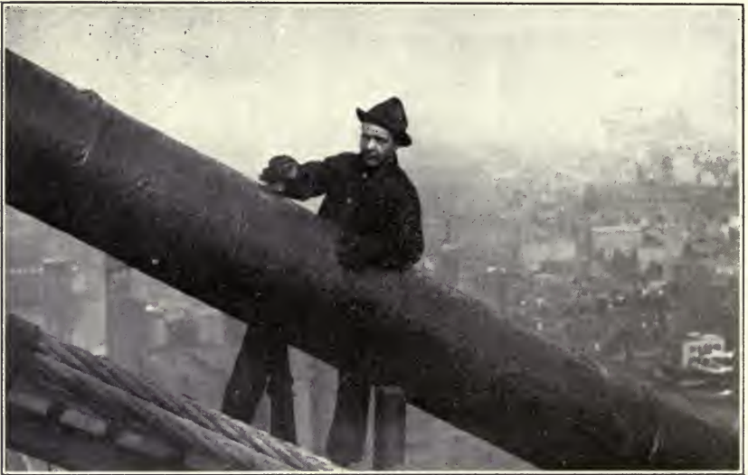
Using a hot iron in cementing the cable coating (design and material from Edw. Smith & Co.) on the Williamsburg Bridge, N. Y. City.
