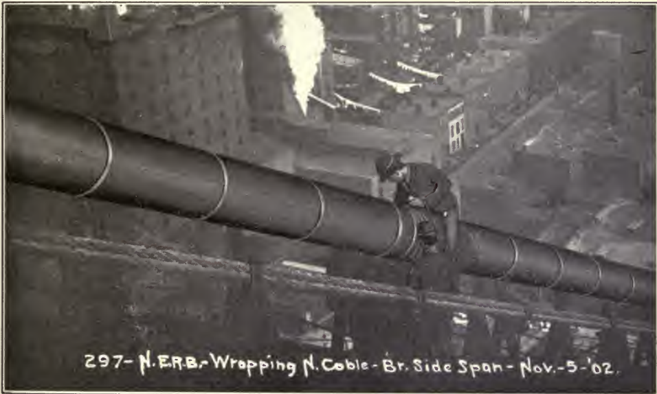
Applying Edw. Smith & Co.'s coating material on cables of Williamsburg Bridge, N. Y. City.
