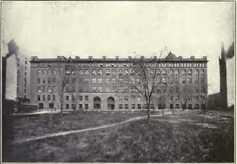
Pierce Building (for engineering), Mass. Institute of Technology. Steel framework painted with Durable Metal Coating.
