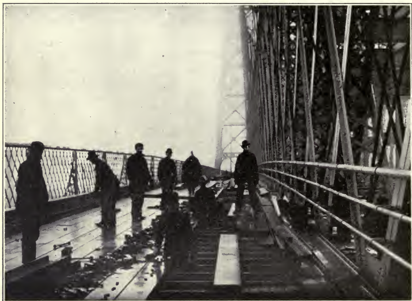
Laying the steel underfloor (coated with Sabin Pipe Coating) on the Williamsburg Bridge, N. Y. City.
