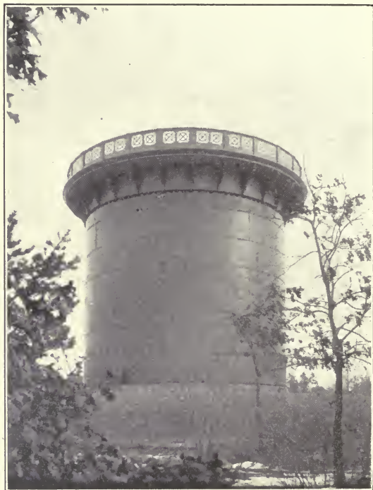
Steel stand-pipe, Winchester, Mass. Height, 40 feet; diameter, 40 feet. This stand-pipe is coated with Durable Metal Coating.
