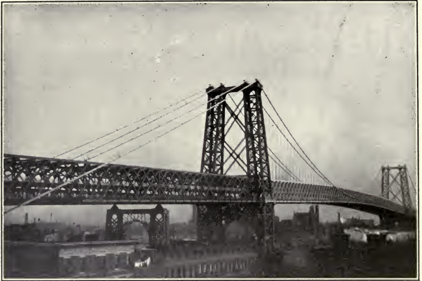
Williamsburg Bridge, N. Y. City. Cables, floor, and anchorage metal work protected with Edward] Smith & Co.'s coatings. L. L. Buck, Ch. Eng. O. F. Nichols, Prin. Asst. Eng.
