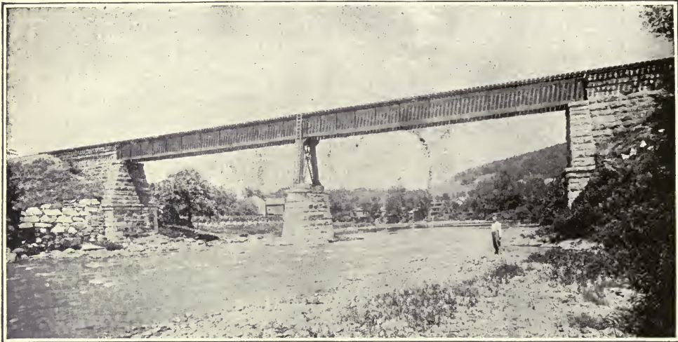
Eagle Bridge, N. Y. Painted with Durable Metal Coating.
