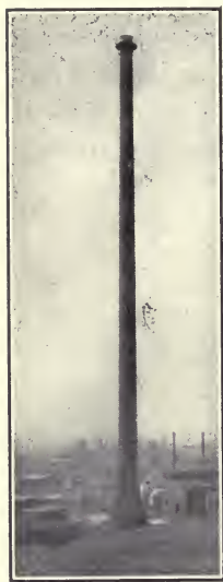
Unlined steel stack, 310 feet high, of the Nichols Chemical Co., Laurel Hill, N. Y. City. This has stood six years, painted on erection with Durable Metal Coating inside and outside, without re-painting.
