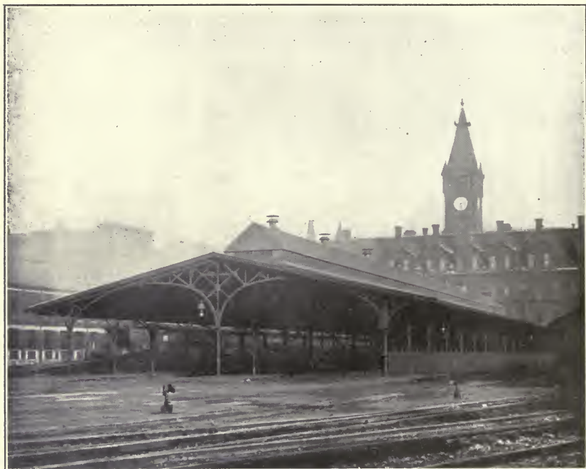
Train-shed of the Wells Street Depot of the C. & N. W. R.R., Chicago. Painted, 1903, with Durable Metal Coating. E. C. Carter, Ch. Eng. W. H. Finley, Prin. Asst. Eng.
