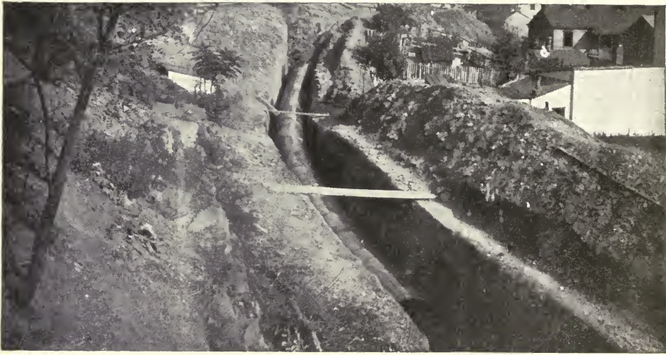
Sixty-inch riveted steel pipe, Allegheny, Pa., 1895. Coated with Sabin Pipe Coating.
