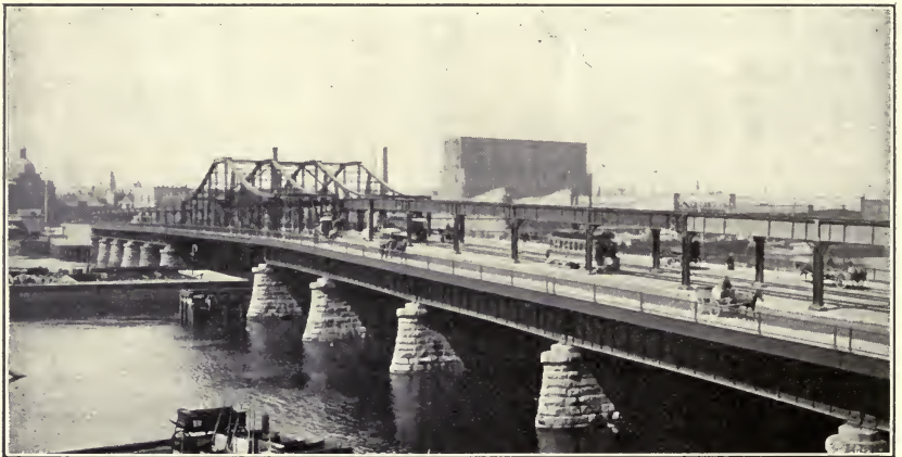
Charlestown Bridge, Boston. Wm. Jackson, City Engr. The girders were painted with Durable Metal Coating, the rest of the bridge with Pelagic] Enamel, made by Edward Smith & Co., N. Y.
