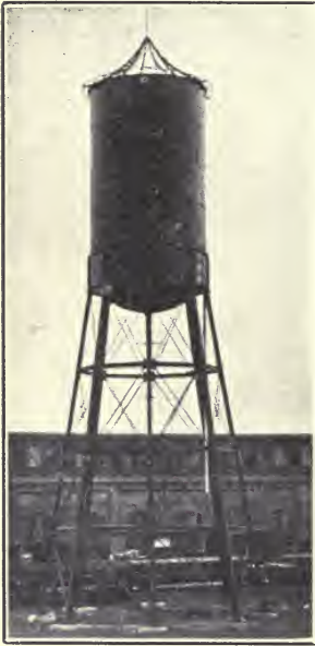
Stand-pipe at Sedalia, Mo., of the M. K. & T. R.R. S. B. Fisher, Cons. Eng. Painted with Durable Metal Coating.
