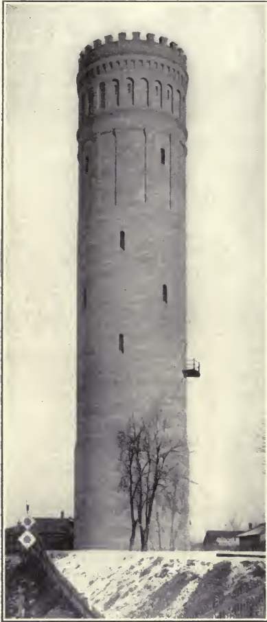
Stand-pipe at Racine, Wis., 135 ft. high. Steel tank painted with Durable Metal Coating. W. H. Laing, Supt.
