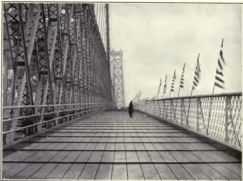
Steel underfloor (coated with Sabin Pipe Coating) ready to receive wood-block pavement, Williamsburg Bridge, N. Y. City.
