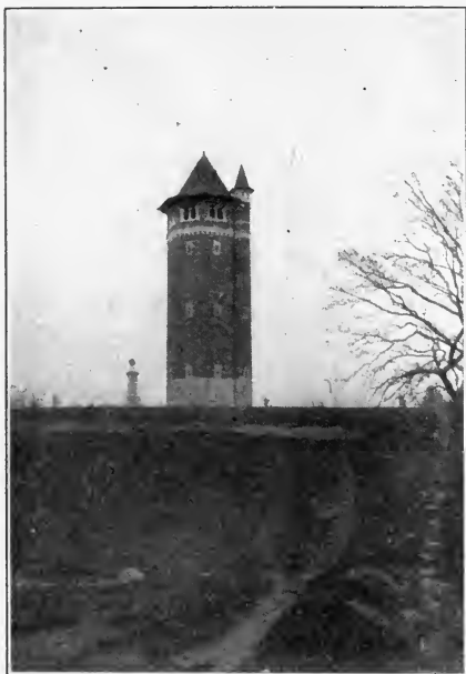
Stand-pipe at Lawrence, Mass. Steel tank painted with Durable Metal Coating.
