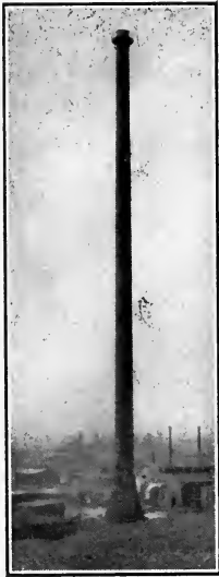
Unlined steel stack, 310 feet high, of the Nichols Chemical Co., Laurel Hill, N. Y. City. This has stood six years, painted on erection with Durable Metal Coating inside and outside, without re-painting.
