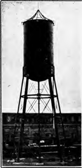
Stand-pipe at Sedalia, Mo., of the M. K. & T. R.R. S. B. Fisher, Cons. Eng. Painted with Durable Metal Coating.
