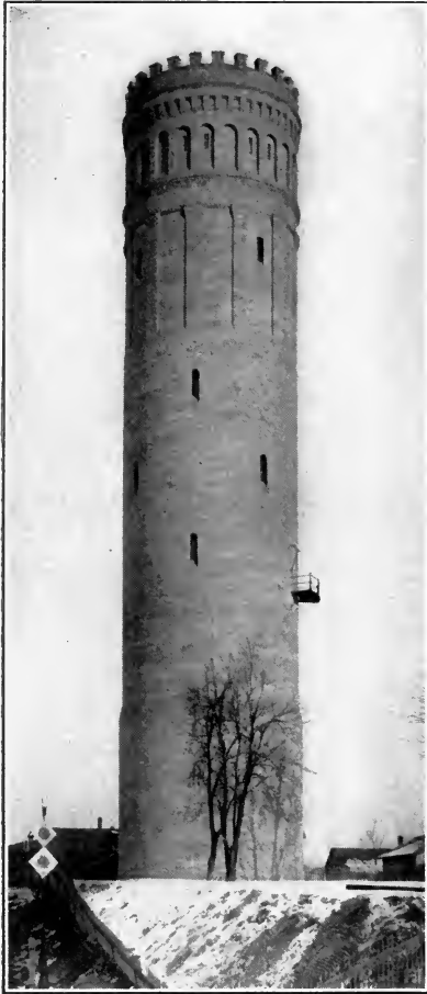
Stand-pipe at Racine, Wis., 135 ft. high. Steel tank painted with Durable Metal Coating. W. H. Laing, Supt.
