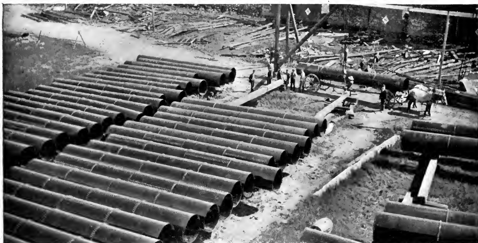
Thirty-eight-inch riveted steel pipe, Rochester, N. Y., 1893. Coated with Sabin Pipe Coating.
