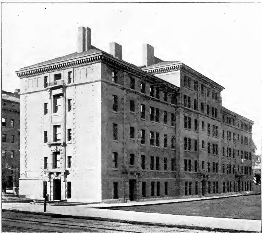
Fayerwether Hall, Yale University. Edward Smith & Co.'s coatings used throughout on this building.
