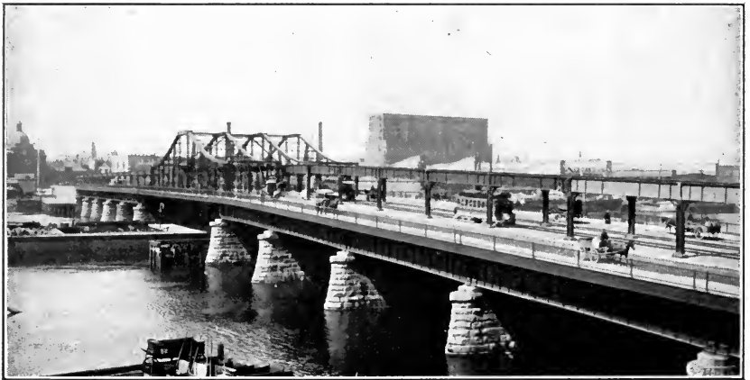
Charlestown Bridge, Boston. Wm. Jackson, City Engr. The girders were painted with Durable Metal Coating, the rest of the bridge with Pelagic Enamel, made by Edward Smith & Co., N. Y.
