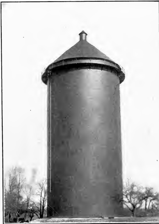
Stand-pipe, Framingham Water Co., South Framingham, Mass. Height, 81 feet; diameter, 40 feet; capacity, 750,000 gallons. This stand-pipe is coated with Durable Metal Coating.
