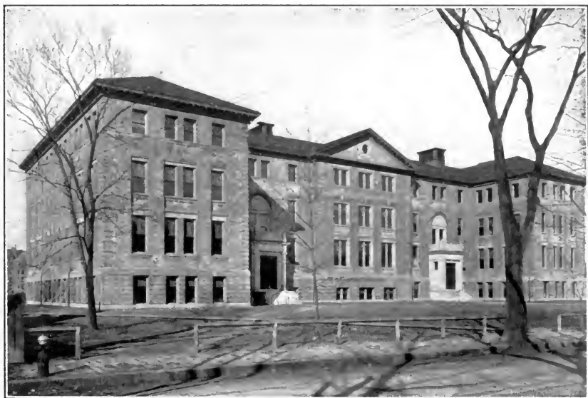
Pierce Hall (Engineering building), Harvard University. Steel framework painted with Durable Metal Coating. Prof. L. J. Johnson, engineer.
