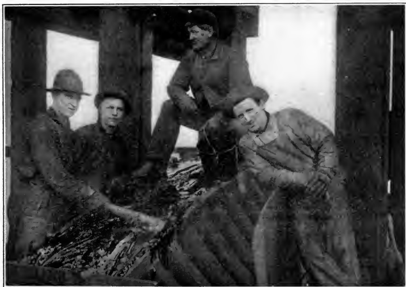
Applying Edward Smith & Co.'s materials on the saddles of the cables of the Williamsburg Bridge.
