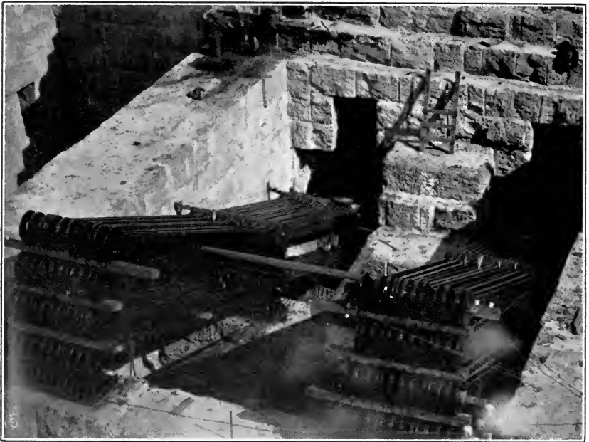
Eye-bar chains in the anchorages of the Williamsburg Bridge. Protected with Ebonite Varnish.
