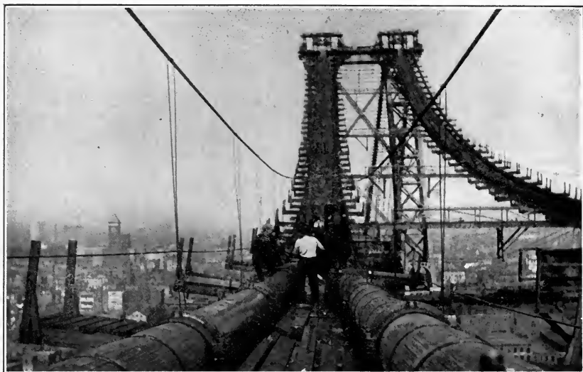
Applying Edw. Smith & Co.'s materials on the cables of the Williamsburg Bridge, N. Y. City.
