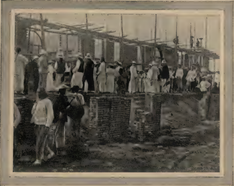
LAYING THE FOUNDATION STONES OF THE NEW COLLEGE.
