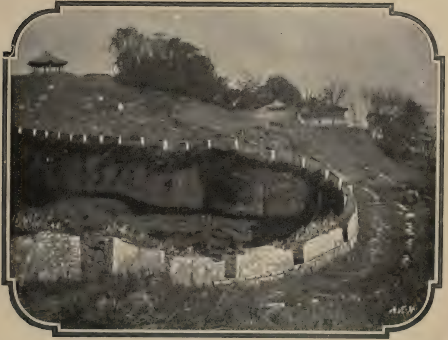
SAN TIEN CITY WALL.
