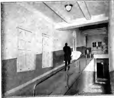
Courtesy Colorado Fuel and Iron Company. INCLINE INSTEAD OF STAIRS IN MINNEQUA HOSPITAL.
