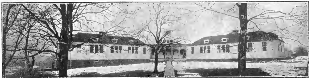
DORMITORY AT DISBROW COLONY, LETCHWORTH VILLAGE.
