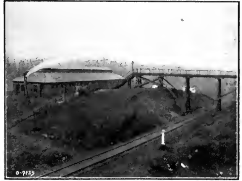
FOR SAFETY AND EFFICIENCY. Change-house and safety over-head walk for employes, Tennessee company.
