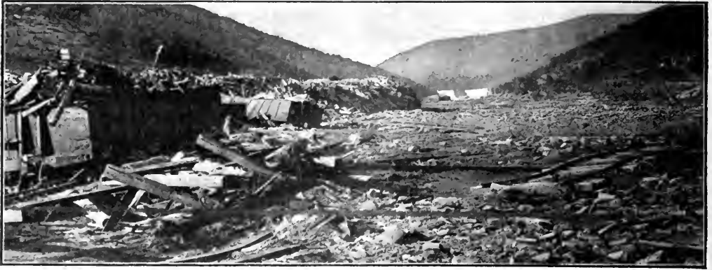
ABOVE AUSTIN—THE BROKEN DAM IN THE DISTANCE.
