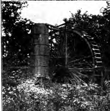
I. Buckets at a spring, Thomas. II. Hand pump and driven well, Republic. III. Old water-wheel pump, and storage tank. [The beginning of a common supply.]
