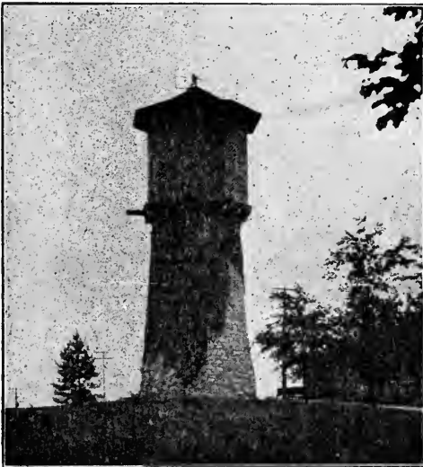
WATER TOWER AT FORT WAYNE, IND.
