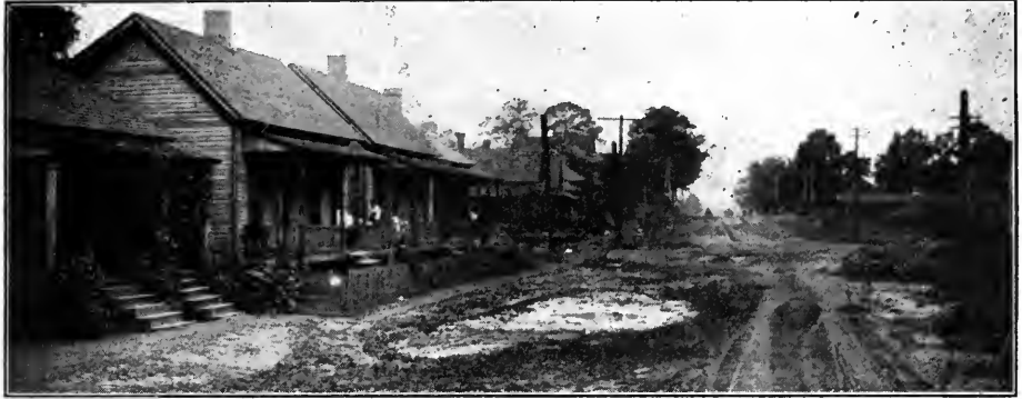
UNSANITARY STREET CONDITIONS, BIRMINGHAM. No drainage, and after every rain the pools become stagnant.
