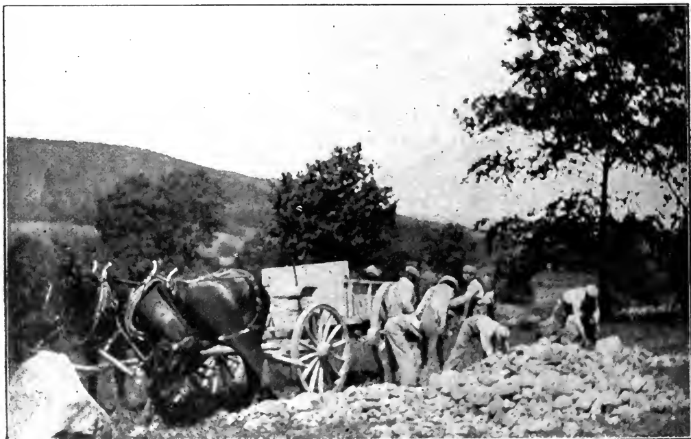
CLEARING LAND FOR PLOWING AT DISBROW COLONY, LETCHWORTH VILLAGE.
