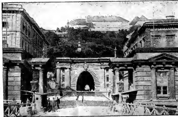
THOROUGHFARE TUNNEL AT BUDAPEST.
