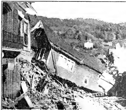
A FRAME HOUSE CRASHED INTO THE TELEPHONE EXCHANGE.
