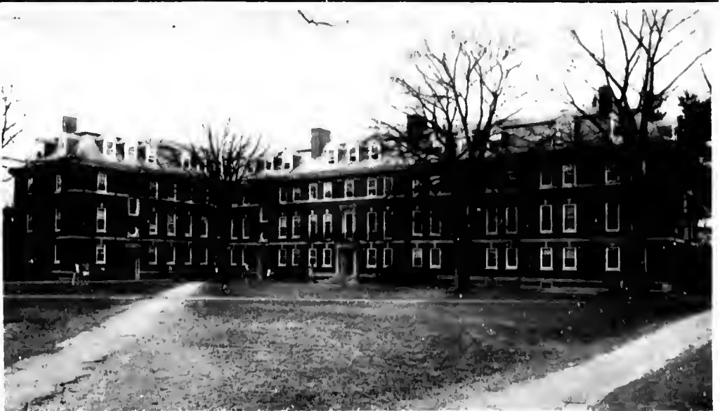
Williams Hall underwent renovations this summer to comply with fire safety regulations. (Buckner)
