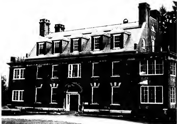
Remodelled Thompson Infirmery is now a home for temporarily displaced students.
