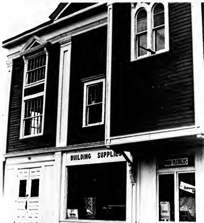
Now housing the Taconic Lumber Company, this building has led a long and varied life. (Burghardt)
