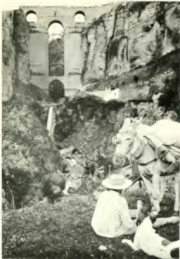
THE FALLS OF THE GUADALEVIN, THE GREAT GORGE AND NEW BRIDGE, RONDA,
