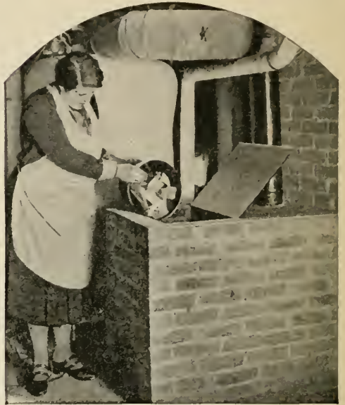
FIG. 22.—All the combustible waste of the household can be burned in this type of incinerator. At the left is shown how the brick walls are laid up after the first grate bars are in place.
