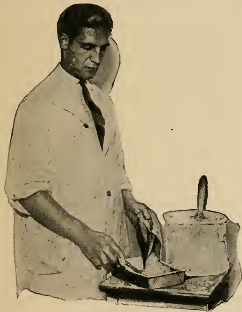
FIG. 26.—Before being added to the plastic paint, the tinting color is mixed into a paste with water.
