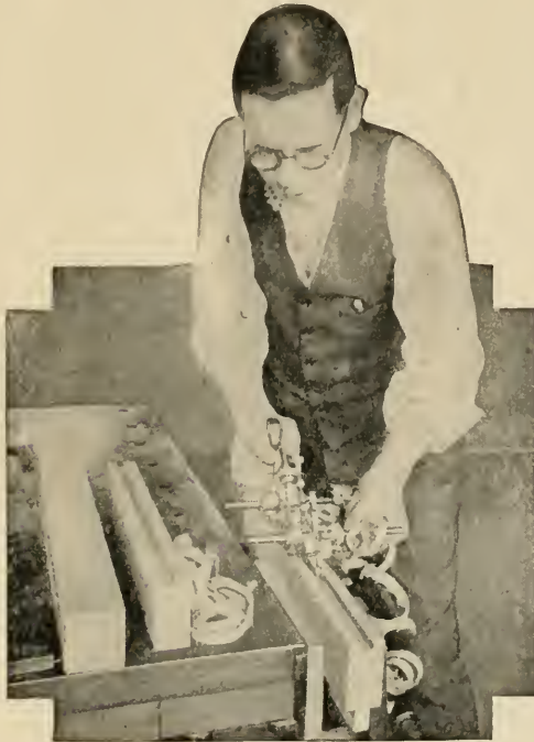
FIG. 13.—Using a combination plane to plow grooves in the rails. Strips can be nailed on instead of making grooves.
