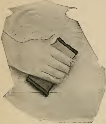
FIG. 20.—For the finest effect on a front door, the enamel is rubbed smooth with pumice stone and water.
