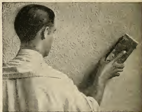
FIG. 30.—Developing a Colonial stipple finish. The brush is known as a painter's "stippling block."
