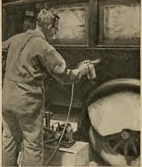
FIG. 4.—The sprayer should be held at about 8 in. from the work and kept in motion at all times.
