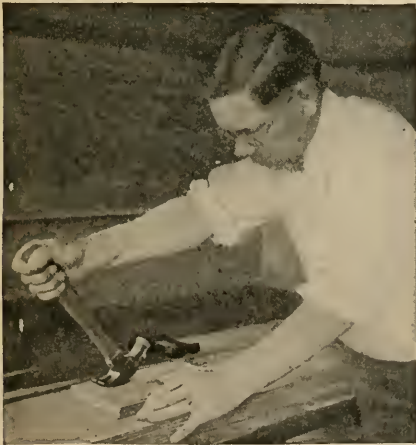
FIG. 10.—The proper way to use a hammer when drawing a nail.
