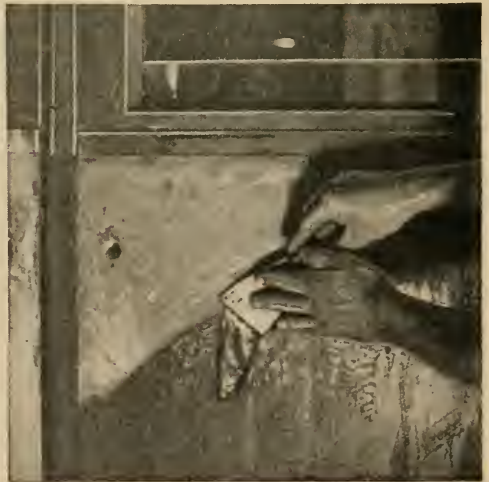
FIG. 2.—Scraping off the old finish. The crinkled finish peels off easily when softened by the remover.
