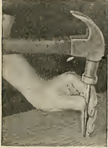
FIG. 13 (right).—Skillful nailing will draw uneven parts into place.
