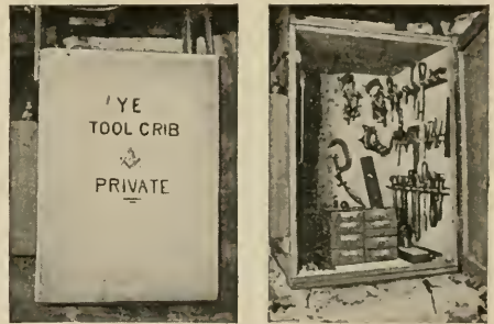
FIG. 24.—This tool cabinet, made from a packing case, is suspended from the first floor beams in the basement.
