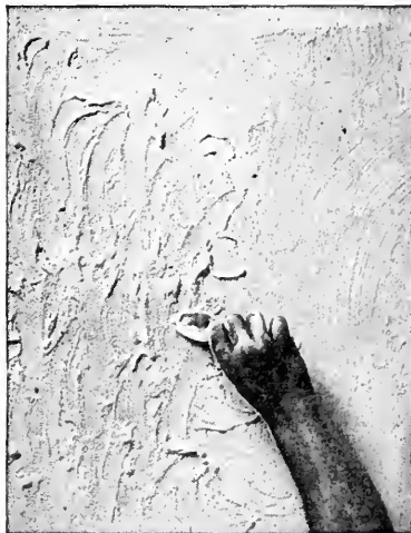
FIG. 27.—The Spanish texture is obtained by stroking the wet paint with the bowl of a common kitchen spoon.
