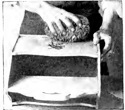
FIG. 18.—The surface is cleaned first with clear water, then with gasoline diluted with water.
