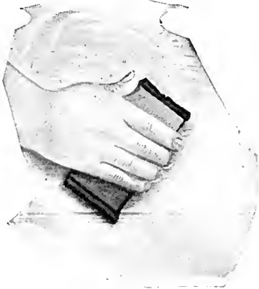
FIG. 20.—For the finest effect on a front door, the enamel is rubbed smooth with pumice stone and water.
