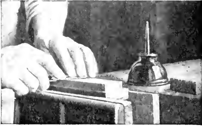
FIG. 11.—When honing a knife, take long strokes back and forth on the oilstone, turning the blade at each stroke and sharpening against the edge. In other words, the cutting edge is pushed forward.
