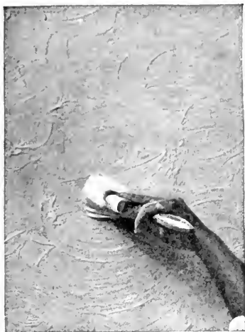
FIG. 28.—Semicircular sweeps of a 4-in. wall brush produce the so-called "monastic" texture.
