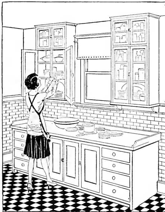
FIG. 10.—A homemade built-in kitchen cupboard with linoleum covered working top. At the bottom is a recess to provide toe space.
