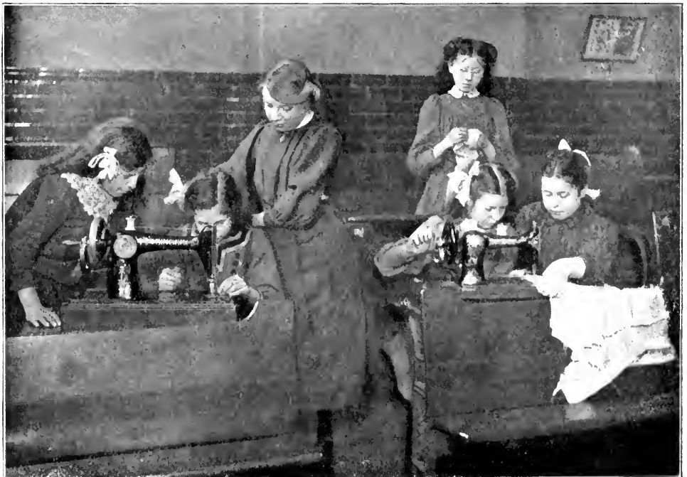
LAWRENCE ROAD COUNCIL SCHOOL
