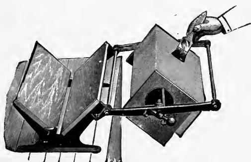
APPLYING THE CEMENT.
