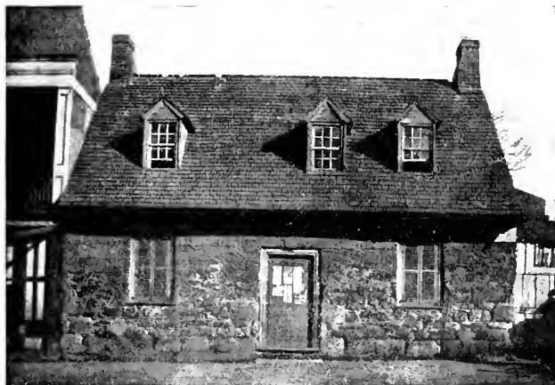
OLD STONE HOUSE, BUILT IN 1737.
