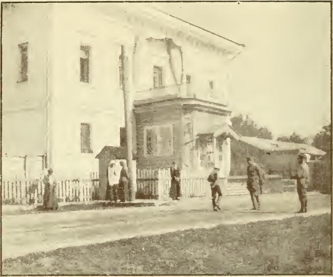
AT THE MAIN DOOR OF THE GOVERNOR'S HOUSE DURING A WALK IN THE COURT.
