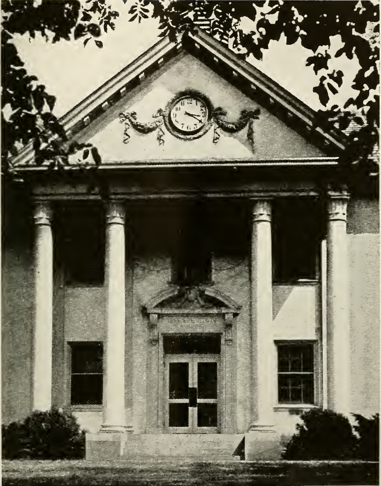
HERBERT D. ALLMAN ADMINISTRATION AND MECHANICS BUILDING
