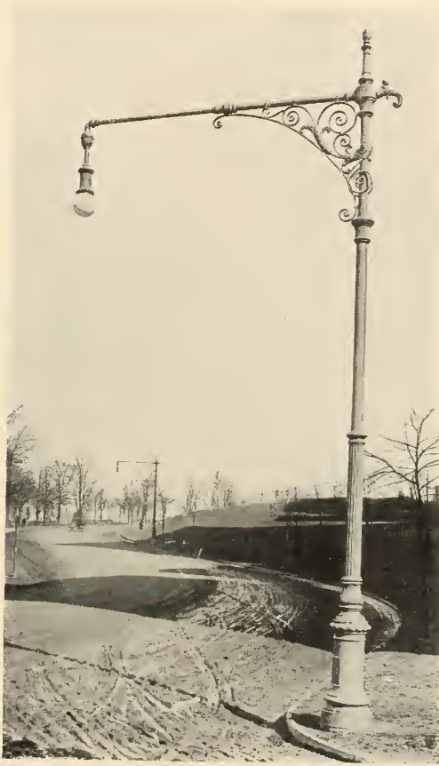
A MAST ARM POST
