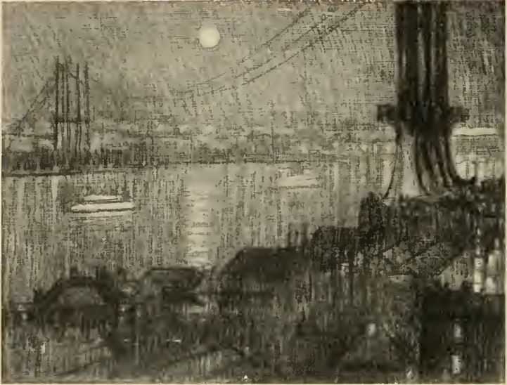
MANHATTAN BRIDGE IN COURSE OF CONSTRUCTION
