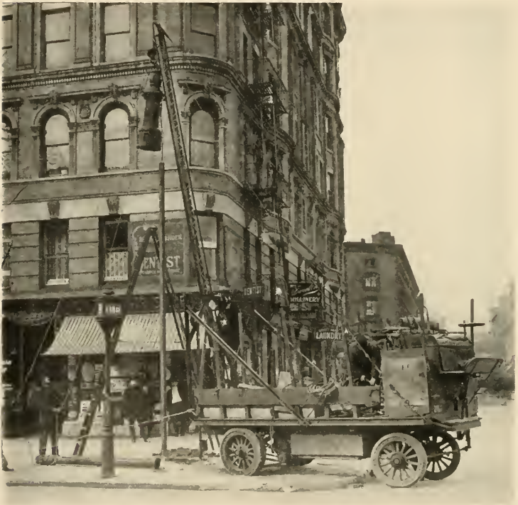
ERECTING A LAMP POST
