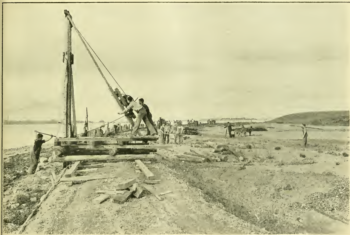
REBUILDING WEST DIKE. VIEW 1.
