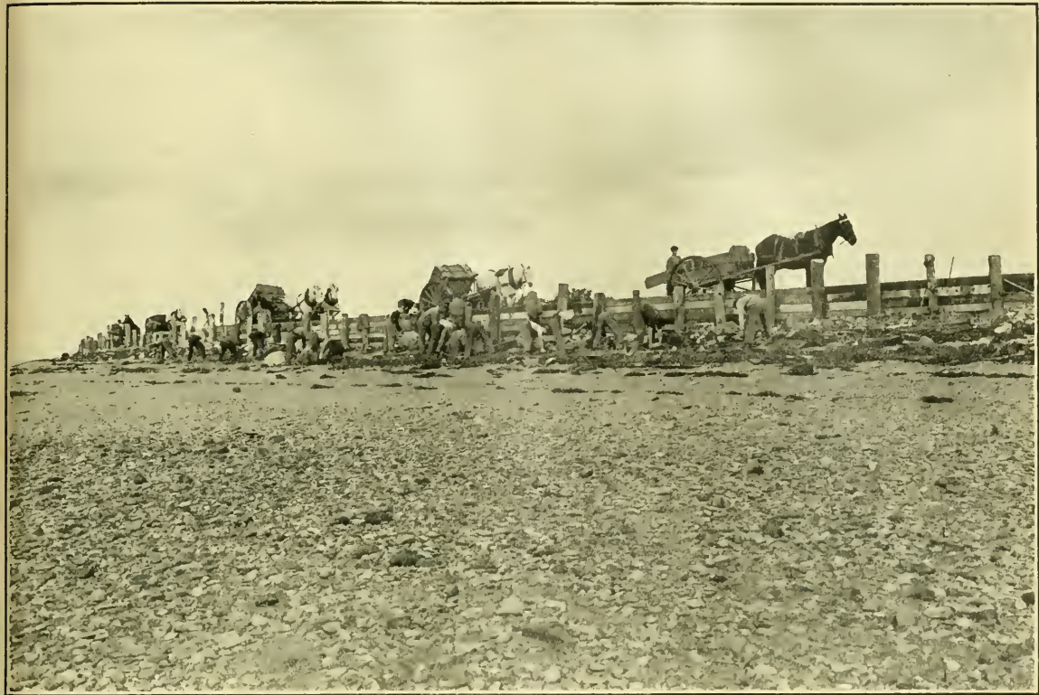
REBUILDING WEST DIKE. VIEW 2.
