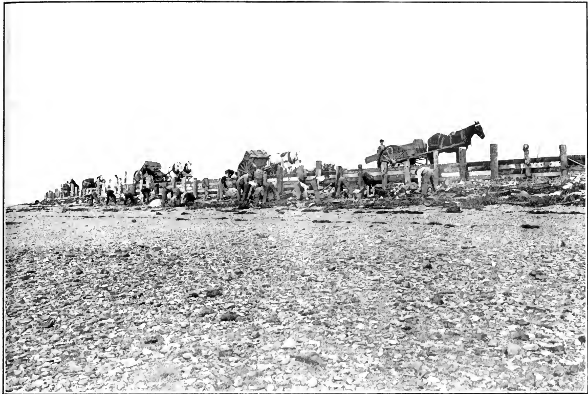
REBUILDING WEST DIKE. VIEW 2.
