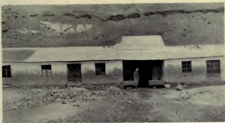
SANTA MARIA: PRINCIPAL ENTRANCE TO THE MINE
