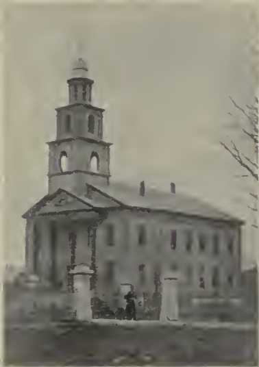
PRESBYTERIAN CHURCH ERECTED IN 1814
