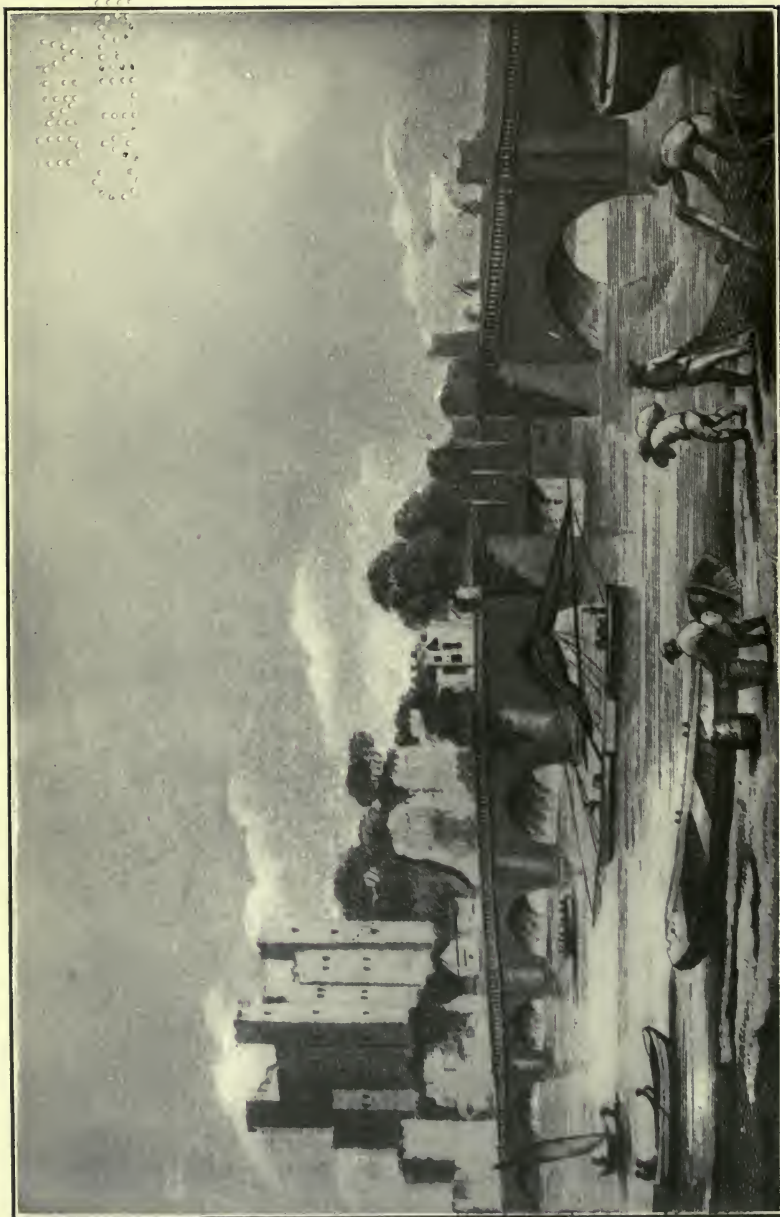
Rochester Bridge, 19th Century (middle arch altered to improve navigation)
