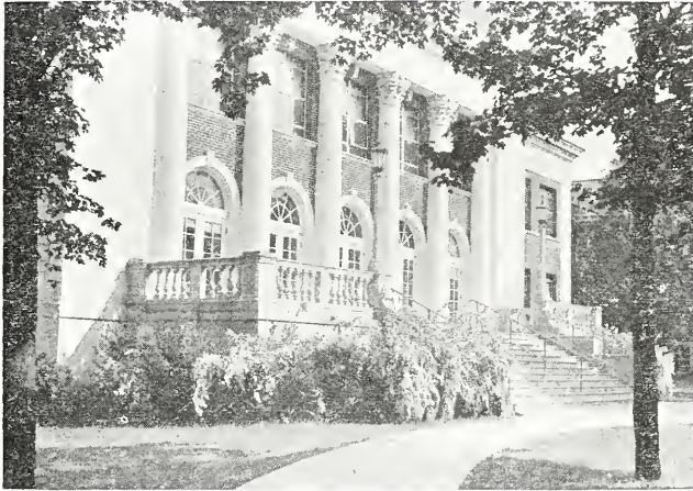
COATES ADMINISTRATION BUILDING
