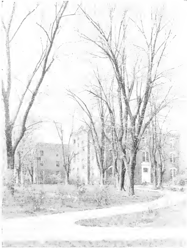
MEMORIAL HALL, MEN'S DORMITORY
