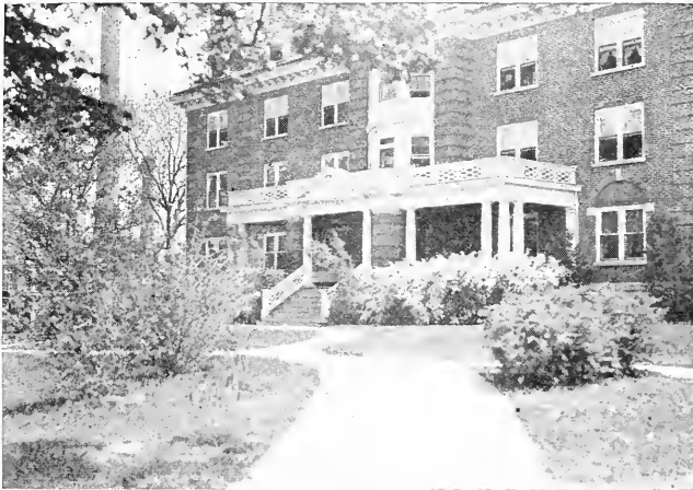
SULLIVAN HALL—WOMEN'S DORMITORY
