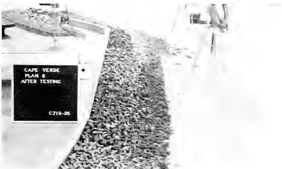
Photo A26. View from north of plan 2 breakwater trunk after testing with 13- and 16-sec, 3.7-m waves
