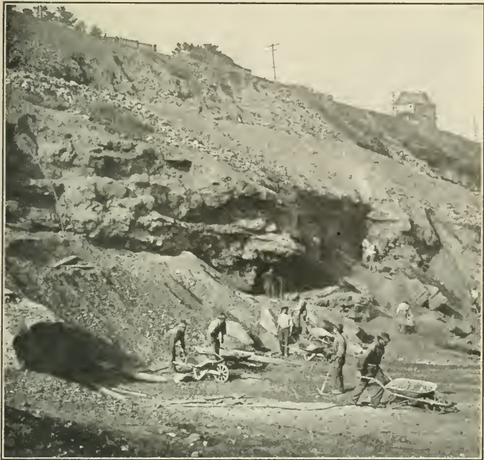
Digging into a seam of coal at the face of a cliff, Pennsylvania.
