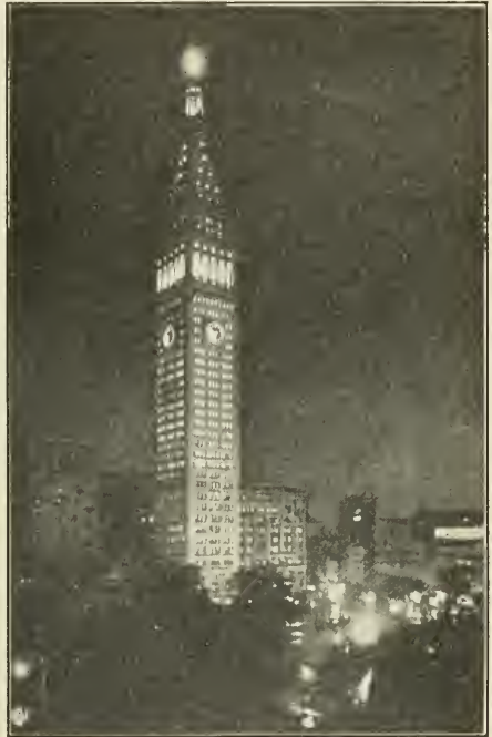
Metropolitan Building, New York.
