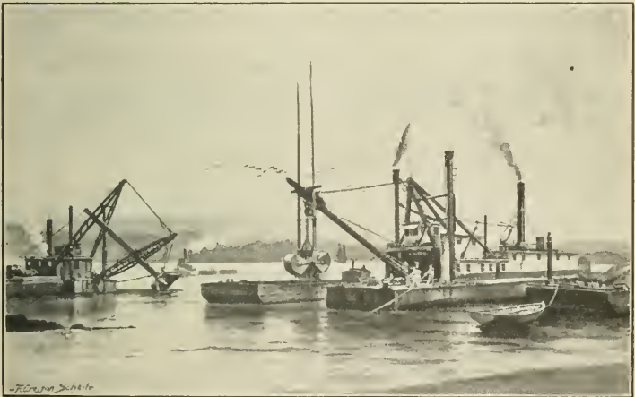
Dredging a river.
