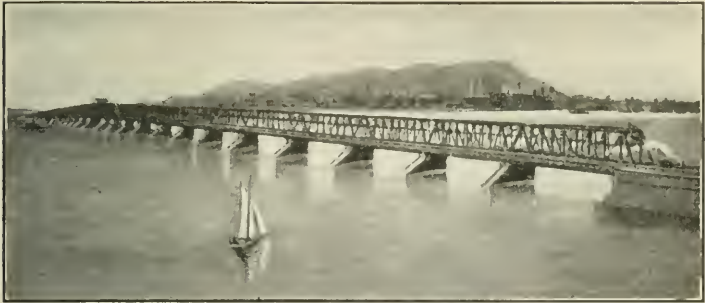
Bridge across the St. Lawrence at Montreal.
