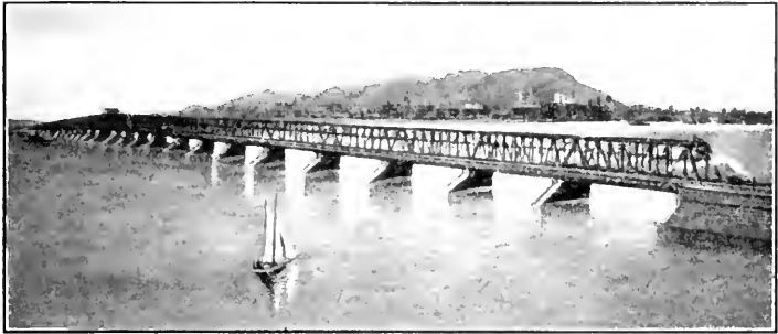
Bridge across the St. Lawrence at Montreal.
