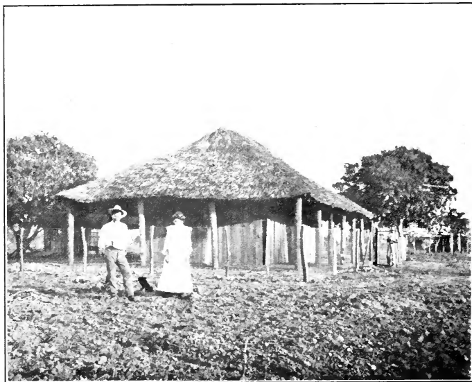
FIG. 4. A Cuban house built for air and coolness, with large thatched roof and clay floor. The trees are mangoes.
