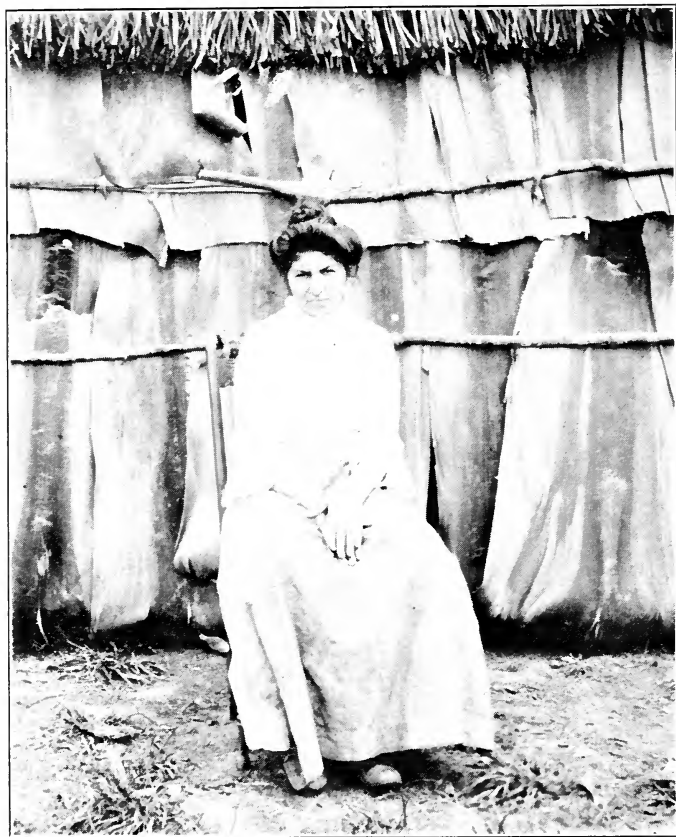
FIG. 35. Leaf-sheaths of the royal palm are often used for the sides of houses.
