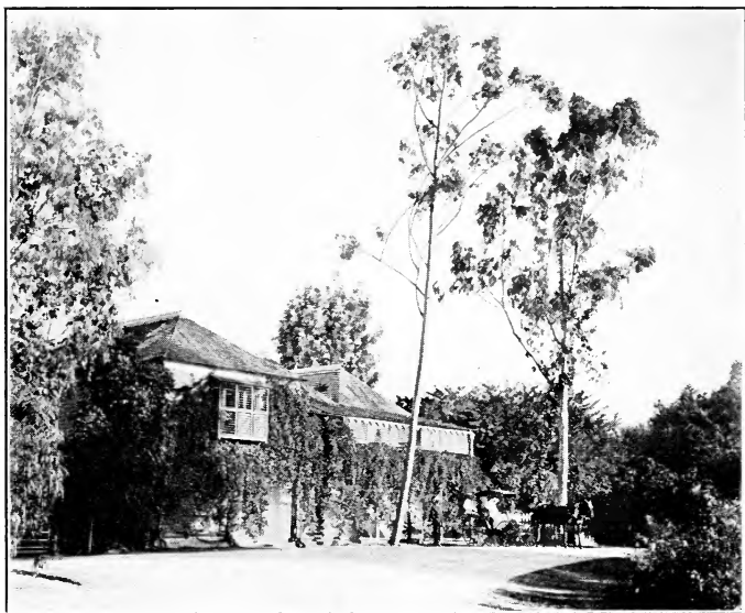
FIG. 70. An attractive tropical house covered with bignonia. The trees are eucalyptus, from Australia, now planted extensively in warm countries because of their exceedingly rapid growth.
