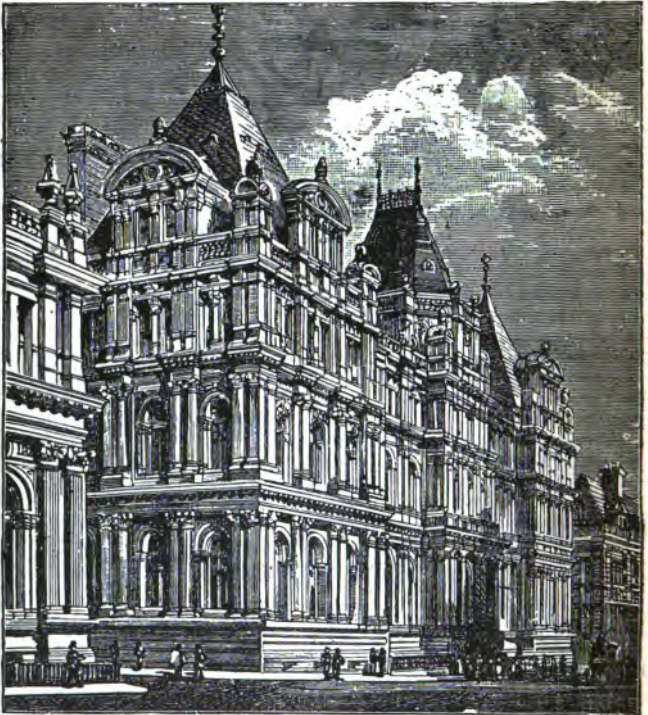
LEEDS MUNICIPAL BUILDINGS.
