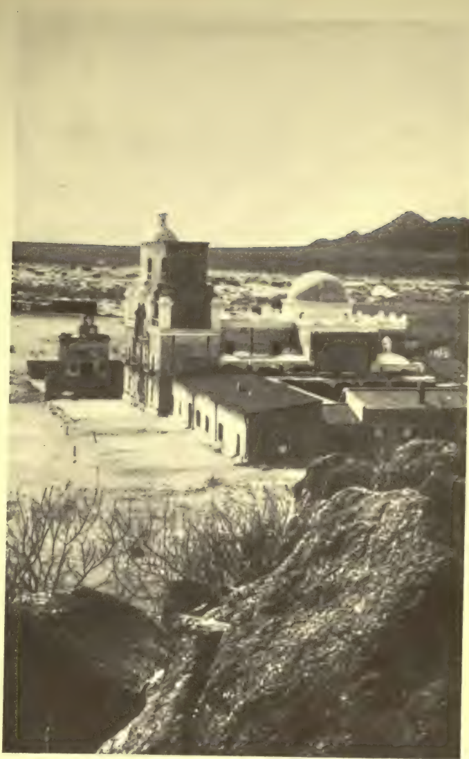
The Mission of San Xavier at Tucson, Arizona, as it was before its restoration
