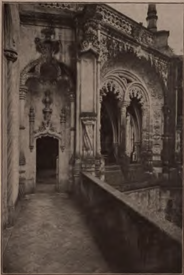
MANUELINE ARCHITECTURE AT THE HOTEL, BUSSACO
