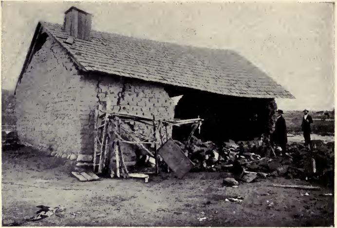
Ruins of adobe house at Saboba that fell and killed several Indians
