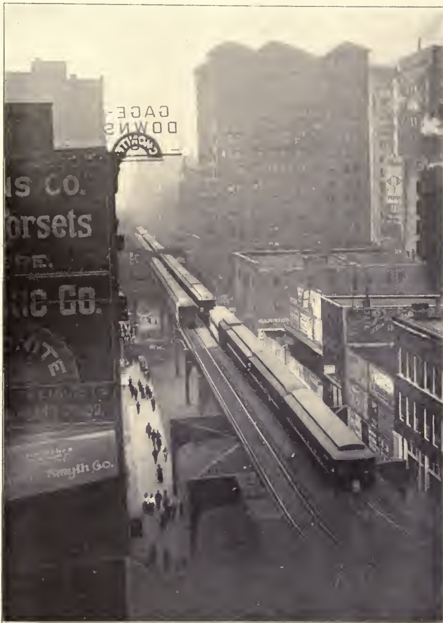
PLATE 25. TRAIN BLOCKADE ON "ELEVATED" LOOP: FIFTH AVENUE, LOOKING NORTH FROM VAN BUREN STREET, 1912.
