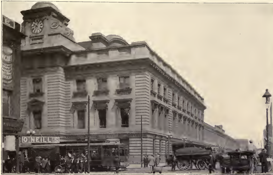
PLATE 49. TERMINAL OF CHICAGO & NORTHWESTERN RAILROAD, CHICAGO.
