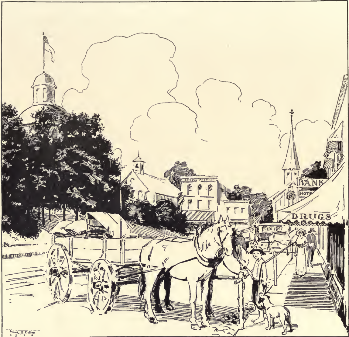
PLATE 28. TYPICAL COUNTRY TOWN HITCHING RAIL.
