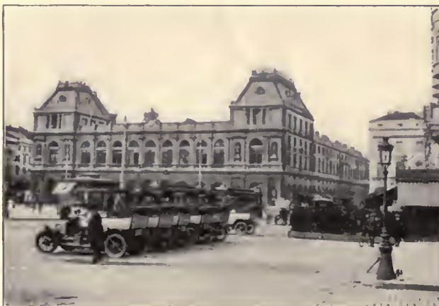
PLATE 34. CAB STAND SPACE AT RAILROAD TERMINAL, BRUSSELS.
