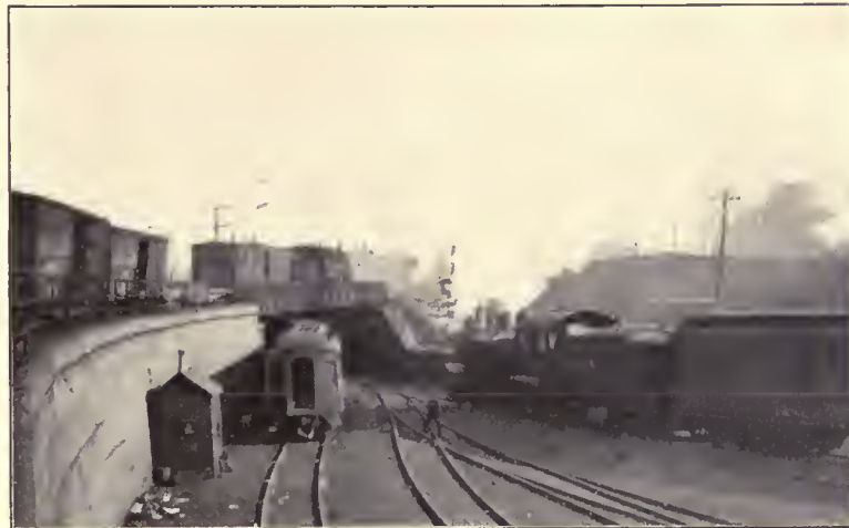
PLATE 15. STEAM RAILROAD CROSSINGS WITH GRADES SEPARATED. ILLINOIS CENTRAL LINE CROSSING OVER ATCHISON, TOPEKA & SANTA FE LINE AT SIXTEENTH STREET AND WENT- WORTH AVENUE, LOOKING EAST. 1914.
