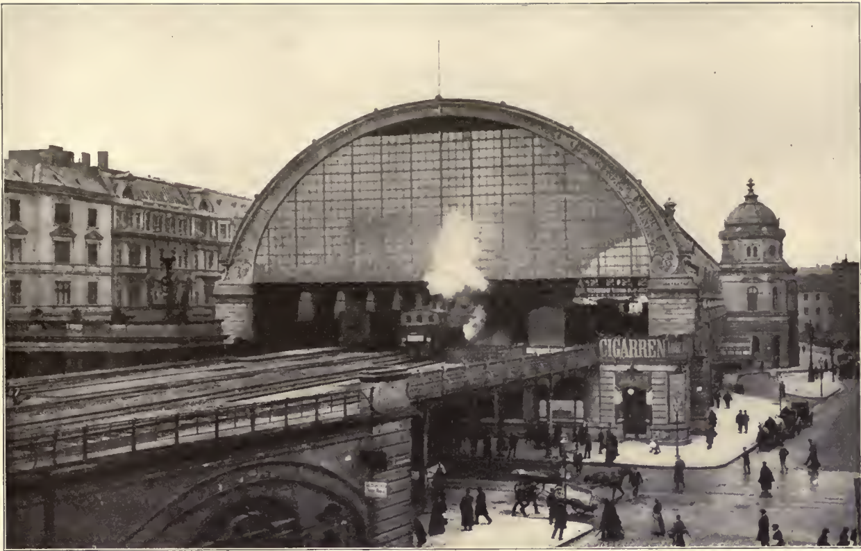
PLATE 61. STATION AT ALEXANDERPLATZ—BERLIN STADTBAHN.
