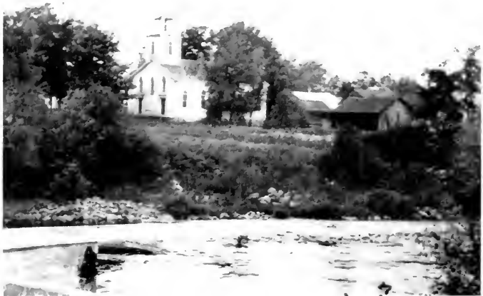
THE BAPTIST MEETINGHOUSE AT FORT COVINGTON, NEW YORK, BUILT IN 1827-29, THE STEEPLE BEING ADDED LATER
