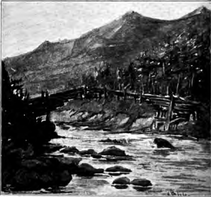
BRIDGE OF SHANG-HO-RI (SOUNDING RIVER) ON THE ROAD TO TANKAR.
