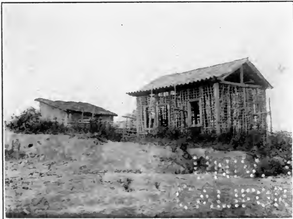
The Frame of a Dwelling House before the Clay Covering is put on.
