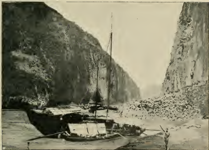
Travelling House-boat, with Tender, moored in Wushan Gorge: Nude Figure in Foreground, Man who swims out to disengage the Tow-lines: Tender is steered by Long Stern-sweep: House-boat with Long Bow-sweep. [To face p. 78.
