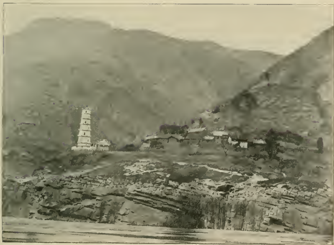
Seven-storied Pagoda below Patung. Note Fluted Rock, about 50 Feet High, on Right Hand, being Ancient "Pot-holes" in the Limestone worn through by the Current (p. 70). [To face p. 70.]
