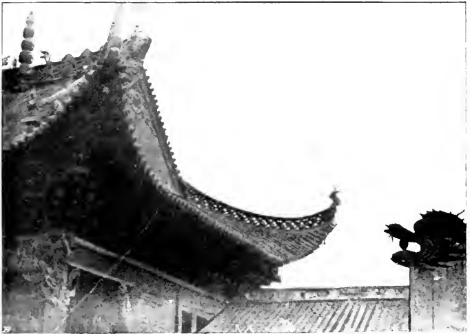
Roof Corner, Guildhall, Chung-king (p. 164).
