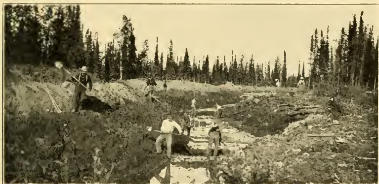
FINISHING THE DITCH.
