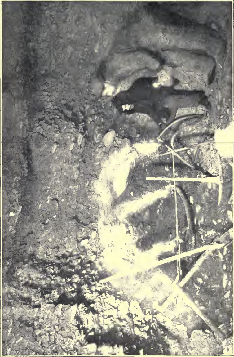
STEAM-POINTS IN PLACE UNDERGROUND.
