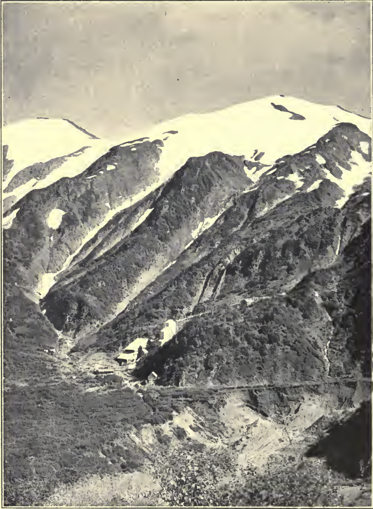
ALASKA PERSEVERANCE MILL IN SILVER BOW BASIN.
