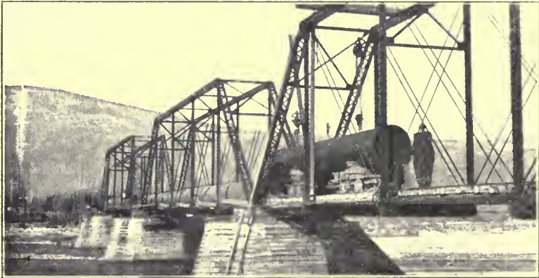
PIPE CROSSING THE KLONDIKE.
