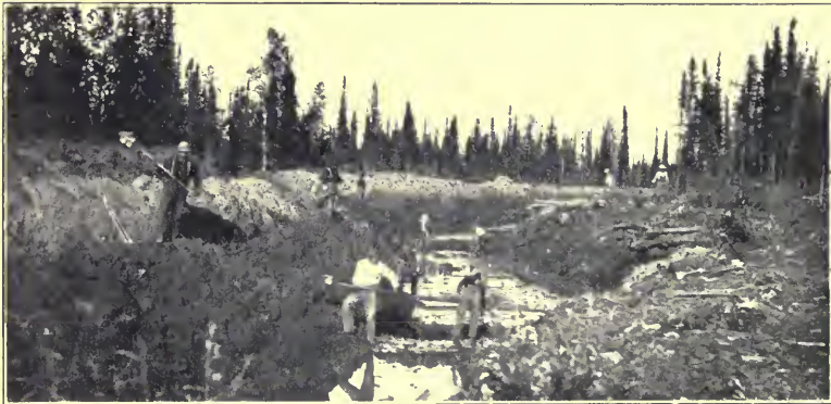
FINISHING THE DITCH.
