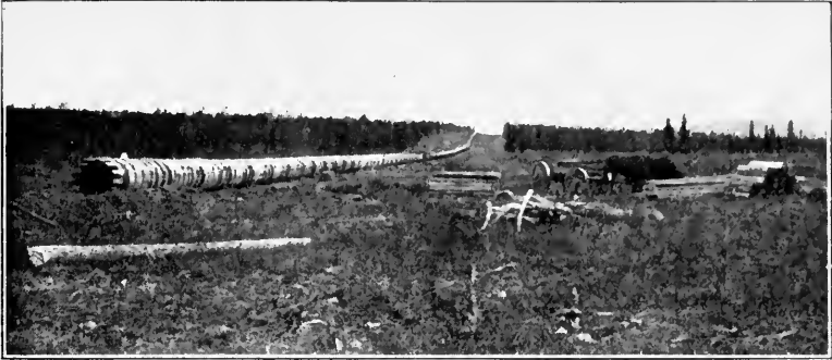
WOODEN STAVE PIPE-LINE.
