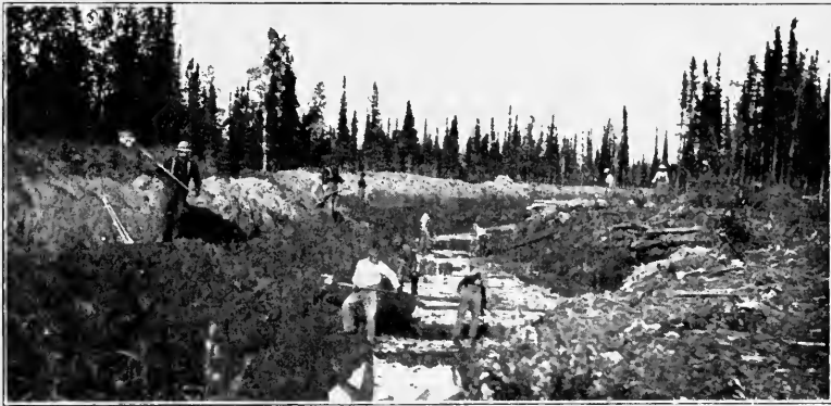
FINISHING THE DITCH.
