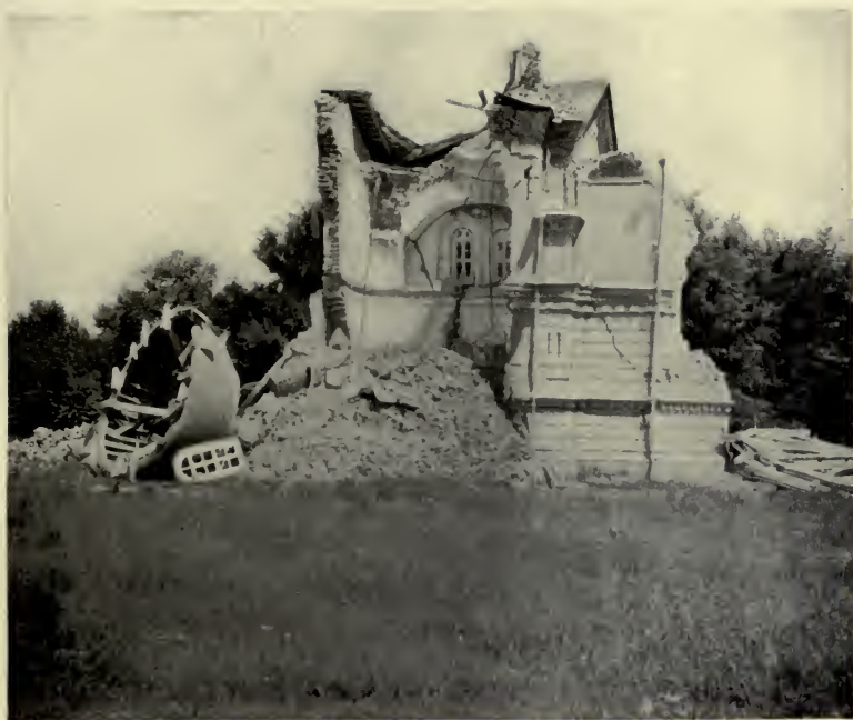
Russian chapel, after the earthquake—Andijan.
