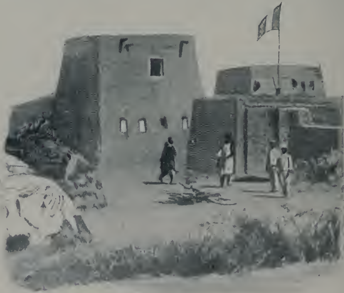
THE FORT OF KABARA
