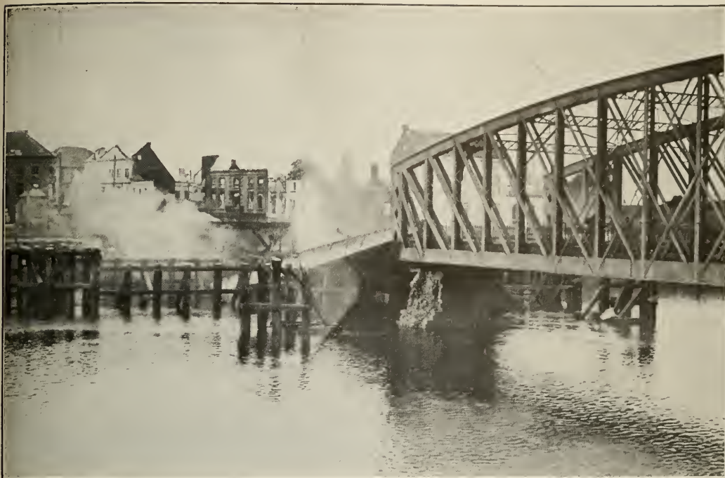
TERMONDE. The Railway Bridge.
