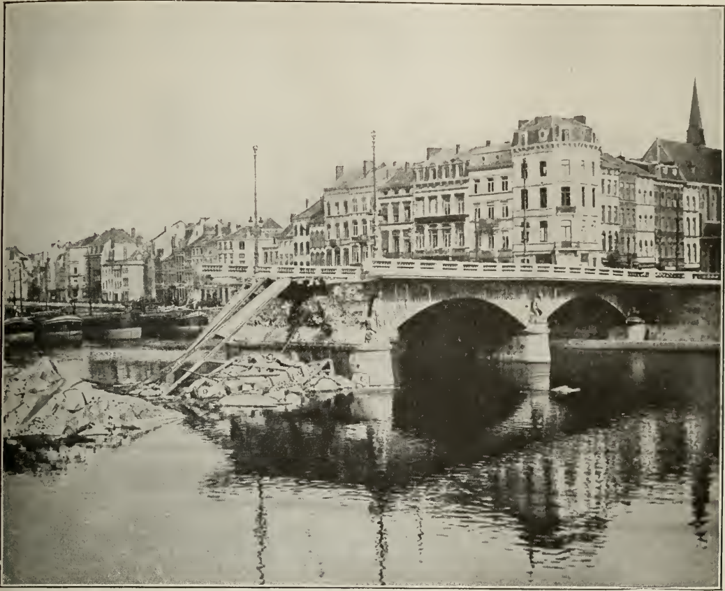
RIGHT SIDE OF BRIDGE AT LIÈGE.
