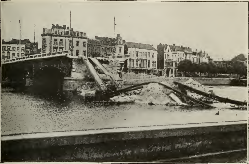
ANOTHER VIEW OF THE RUINED BRIDGE.
