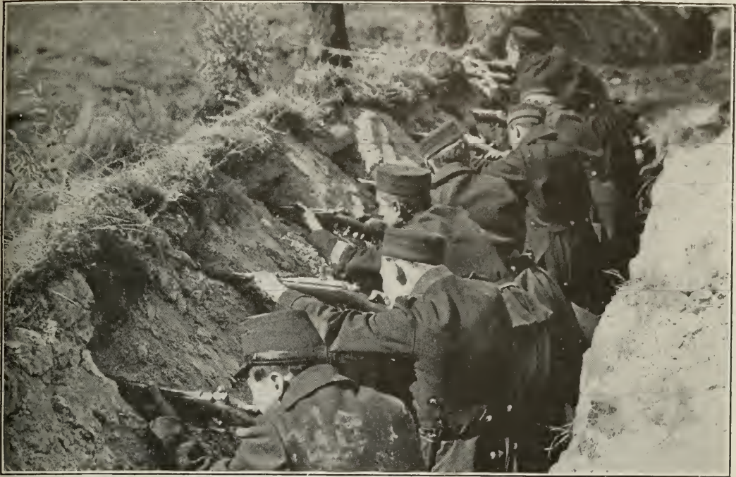
INSIDE A BELGIAN TRENCH.
