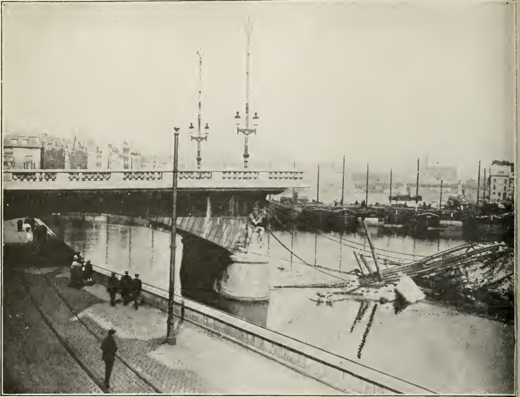
LEFT SIDE OF THE FAMOUS BRIDGE AT LIÈGE. Blown up by Belgians to impede the German Advance.
