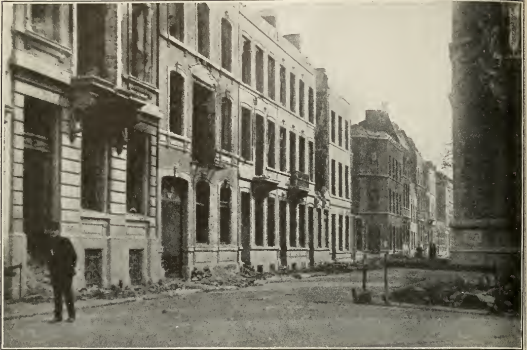
A RUINED STREET IN LIÈGE.
