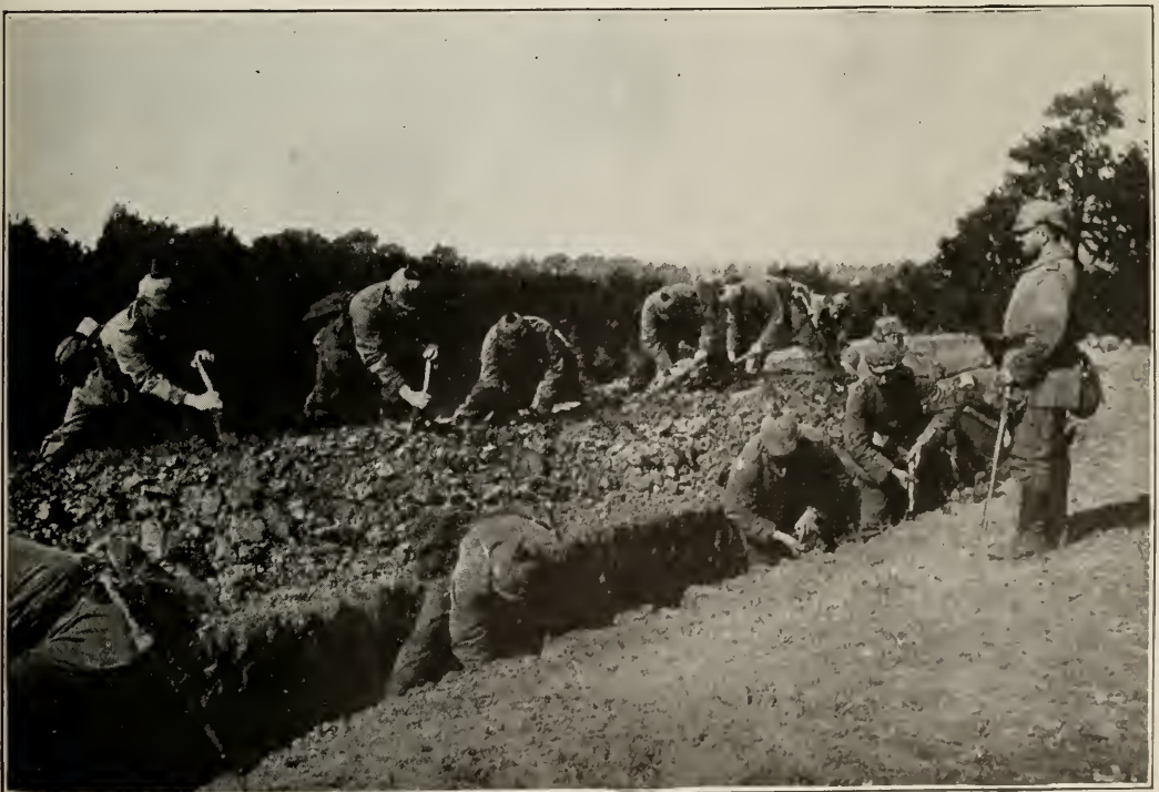
A GERMAN SHELTER TRENCH.
