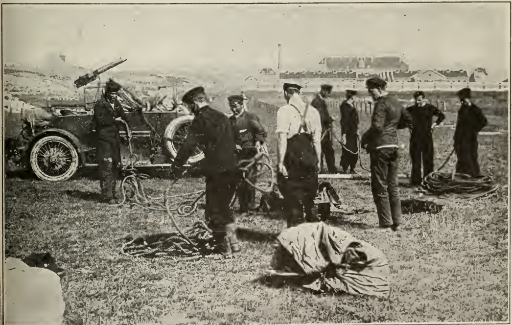
A SECTION OF THE ROYAL FLYING CORPS AT THE FRONT.
