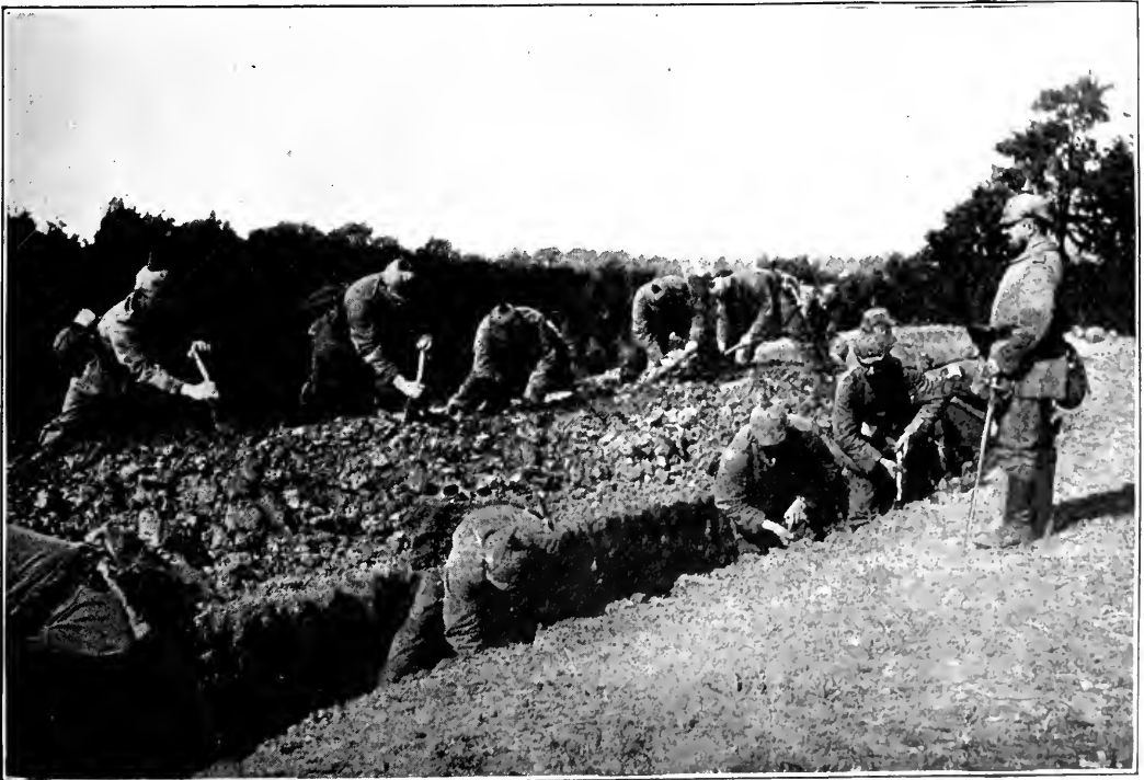
A GERMAN SHELTER TRENCH.
