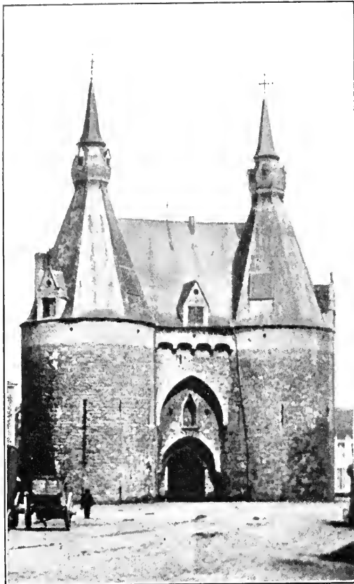
MALINES. The Old Brussels Gate.
