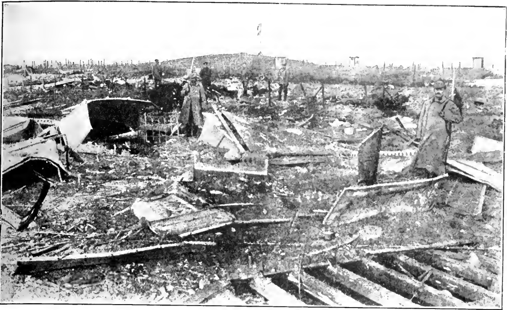
GROUND SURROUNDING ONE OF THE LIÈGE FORTS.
