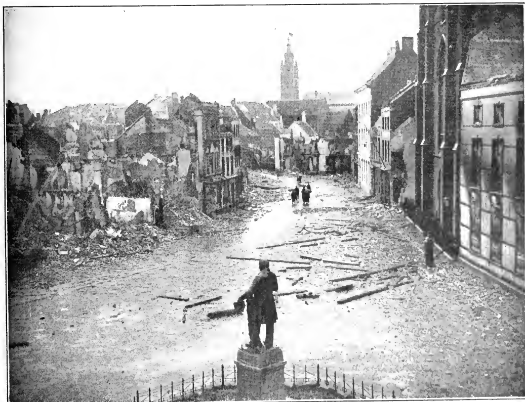
TERMONDE. Scene of Destruction.
