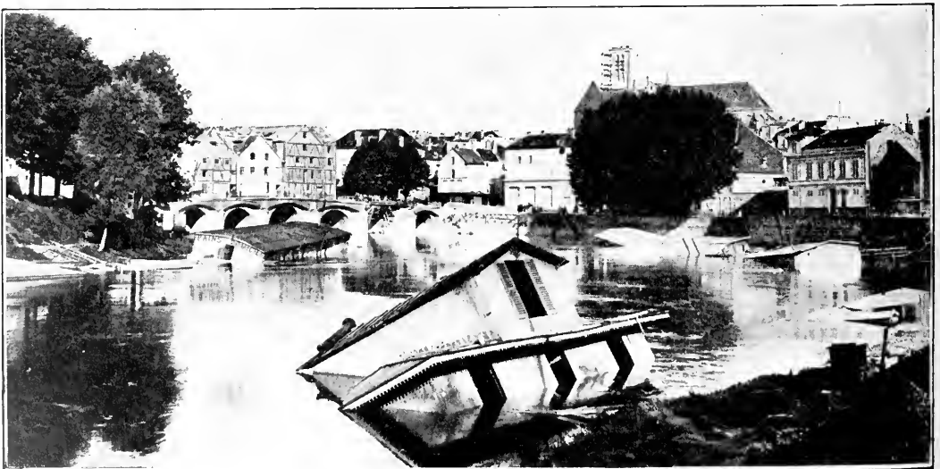
MEAUX FROM THE RIVER MARNE. Showing the broken bridge and sunken house-boats.
