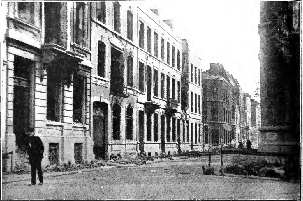
A RUINED STREET IN LIÈGE.
